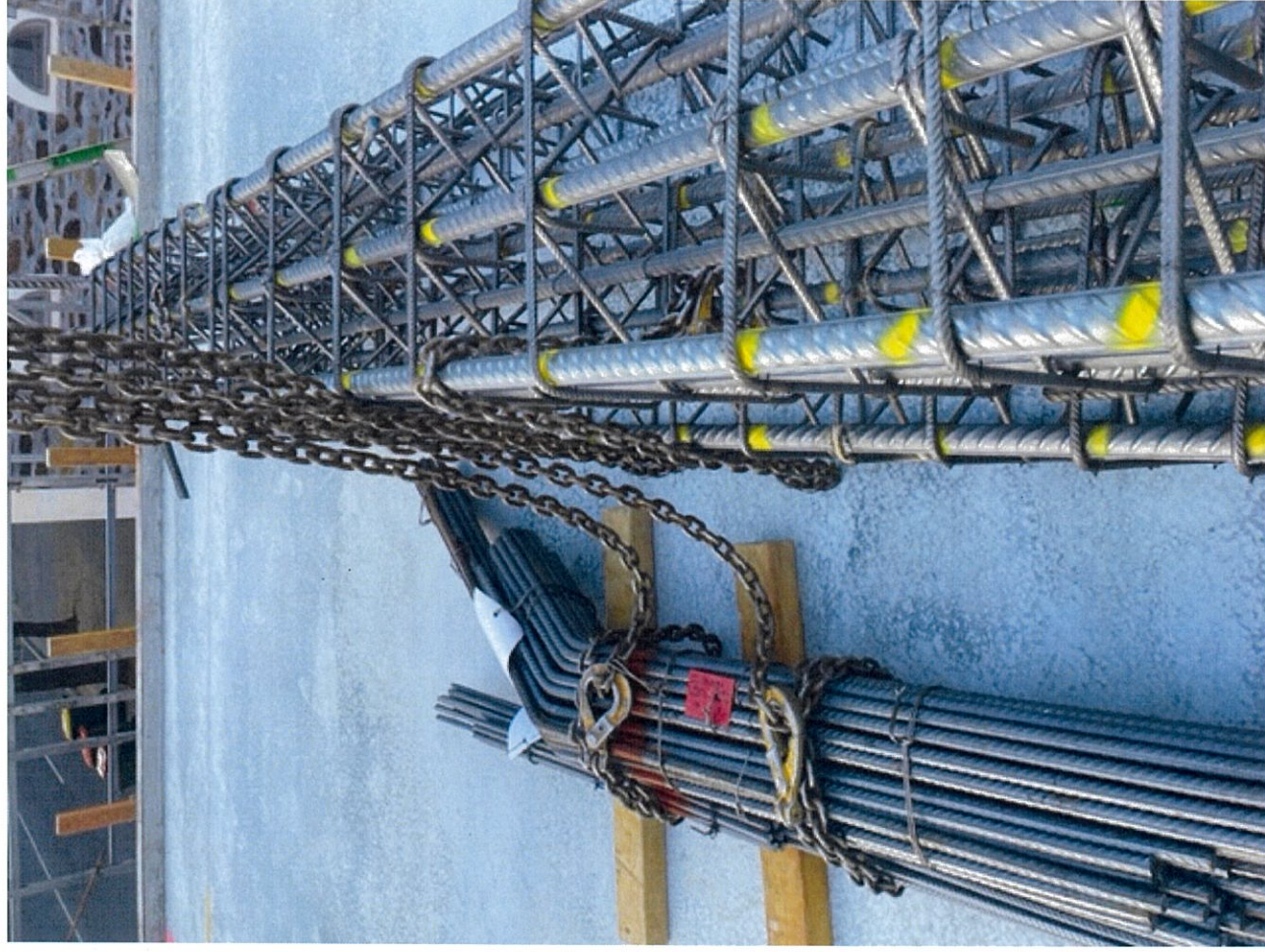
The two reo bar loads slung in the recent incident.
