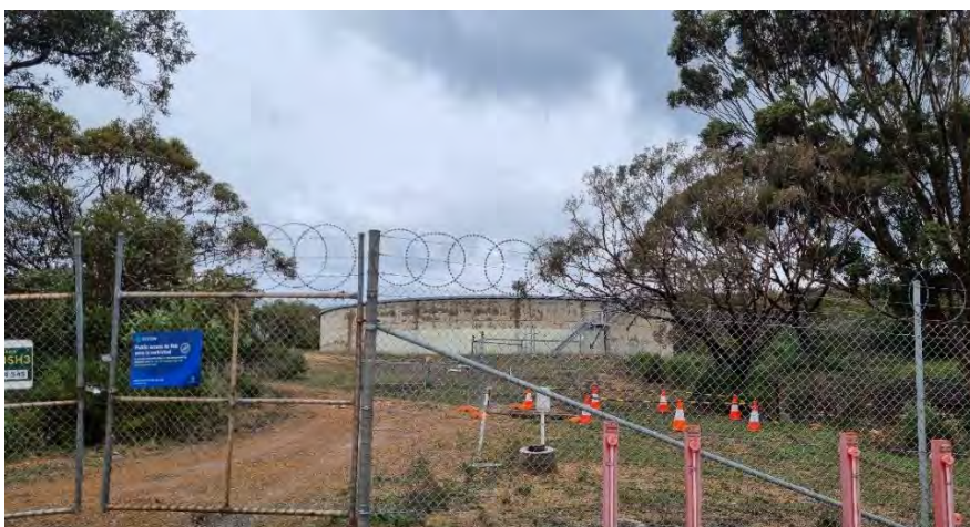
Figure 7.8 North Side Hill Tank site
