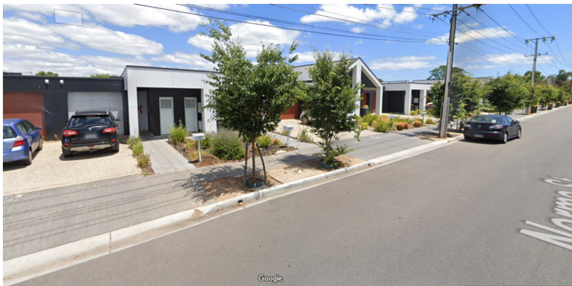
Image 4: Street view of development at Norma Street, Mile End
