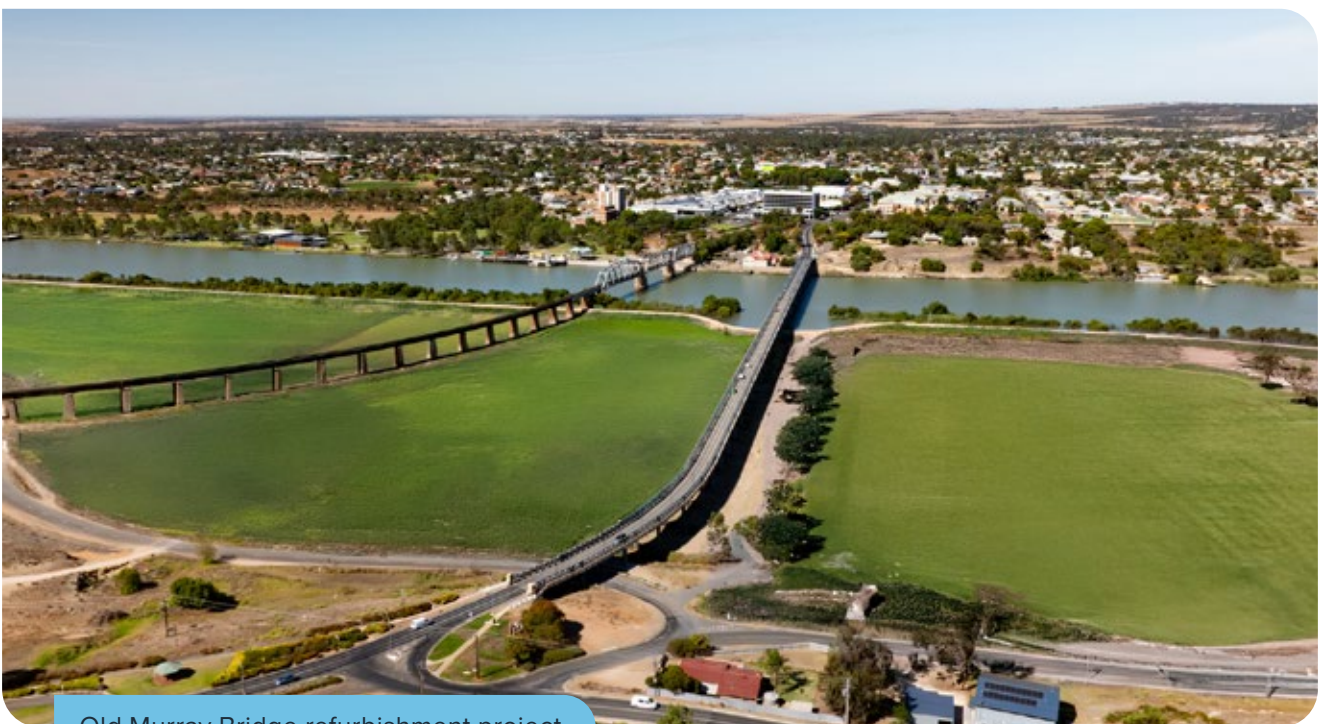
Old Murray Bridge refurbishment project
