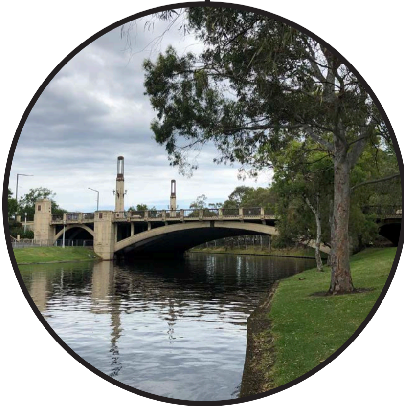
ADELAIDE BRIDGE OVER RIVER TORRENS
