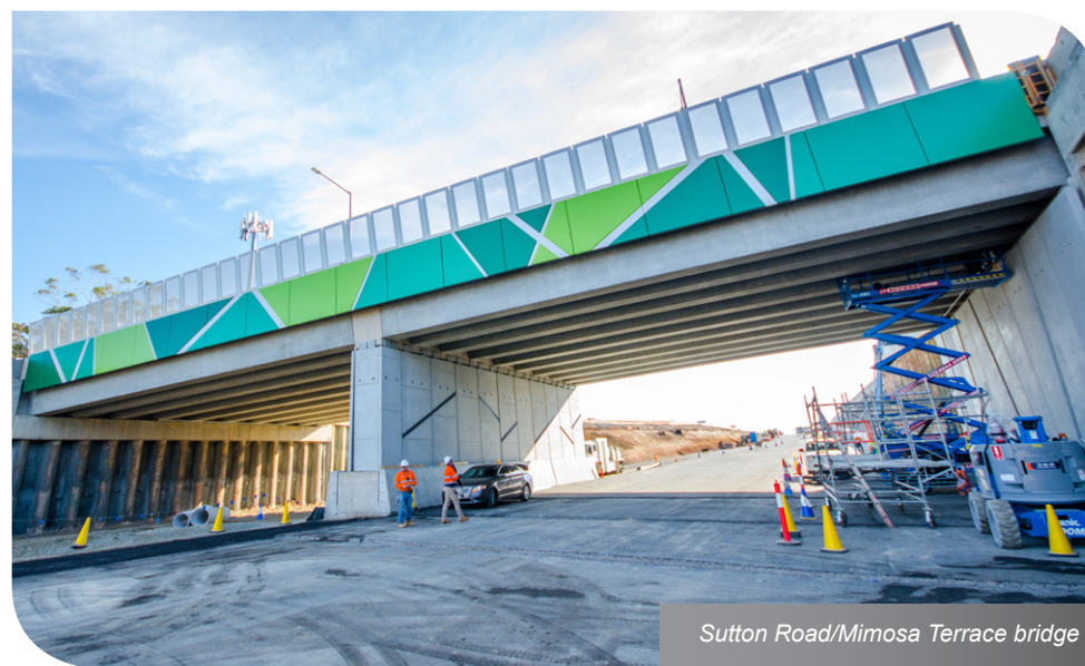
Construction of the Tonsley Boulevard bridge
