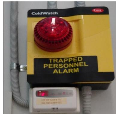
*Recently retro-fitted "Trapped Personnel" alarm that flashes is located externally above the cool room door.*
