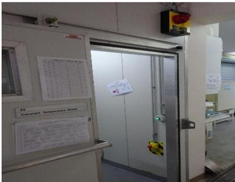
*External view of cool room showing compliant internal light switch and duress button.*
