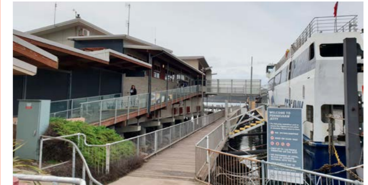
Ferry terminal (left), main jetty access (middle) and ferry wharf (right) as viewed from land.
