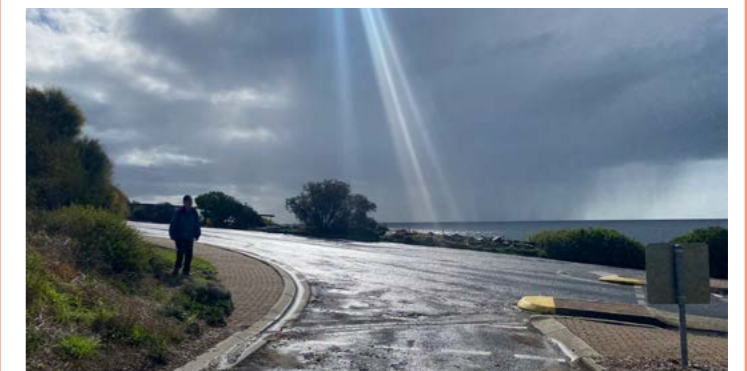
One-way car lane from Bay Terrace to the car marshalling area. Poor sight lines.
