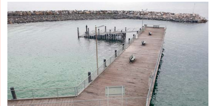
Jetty, with seating and mooring for cruise ships.
