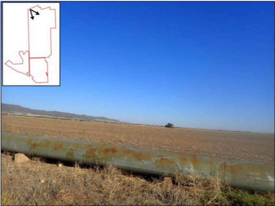
Figure 3 - Site Photo (Source: EPS Energy, Nov 2018)
