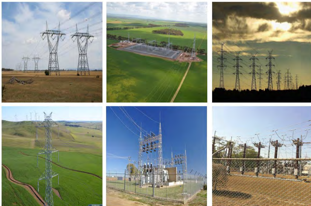
Figure 2-5: Existing Electrical Infrastructure in Australia
