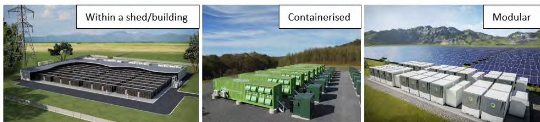
Figure 4-4: Examples of Utility-scale battery Technology Options
