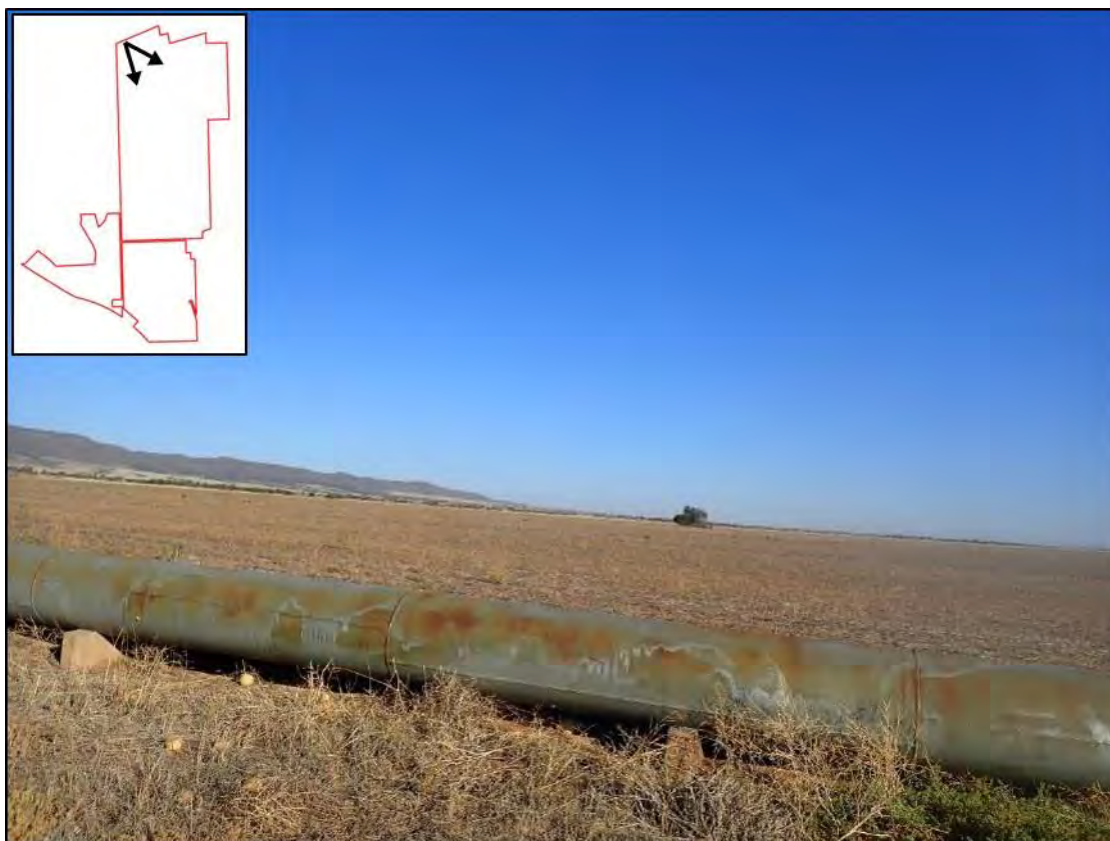
Plate 2: Flat Terrain on Project Area, Morgan-Whyalla Pipeline Along Gulf View Road
