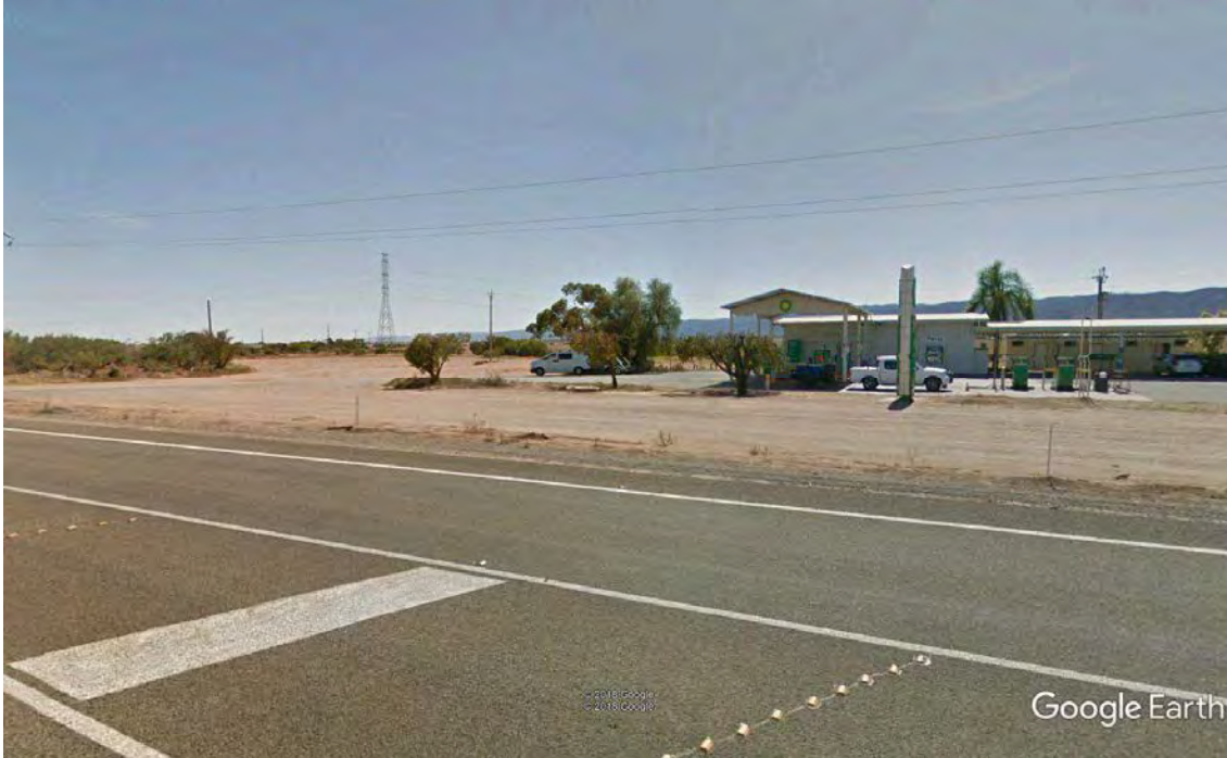
Figure 16: OP04 Warnertown Road Petrol Station looking NORTH
