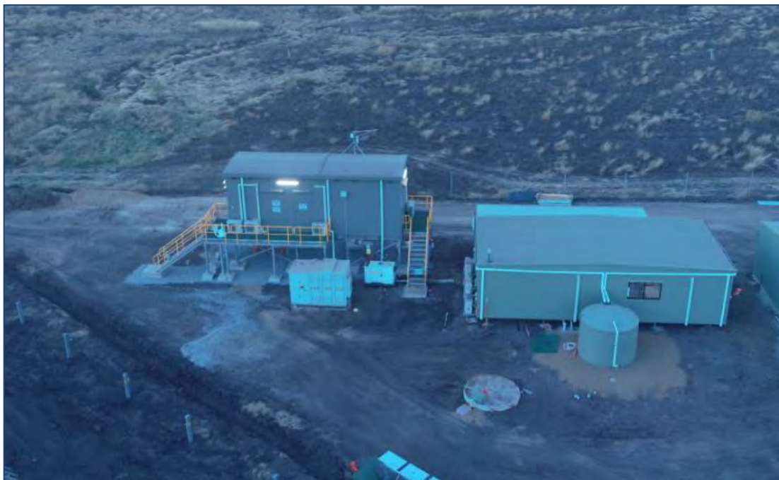
Figure 4-8: Example of a Typical Switch Room-Alongside O&M Building
