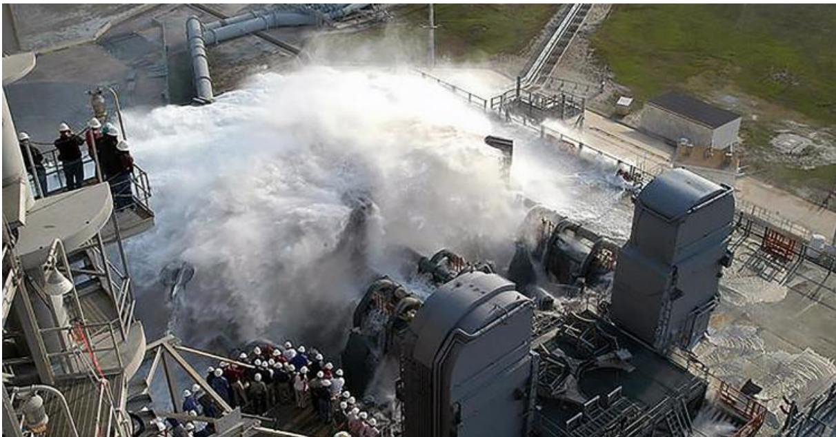
Figure 9 Kennedy Space Centres Launch Pad 39A water sound suppression system (NASA - https://www.nasa.gov/missions/shuttle/f_watertest.html )
