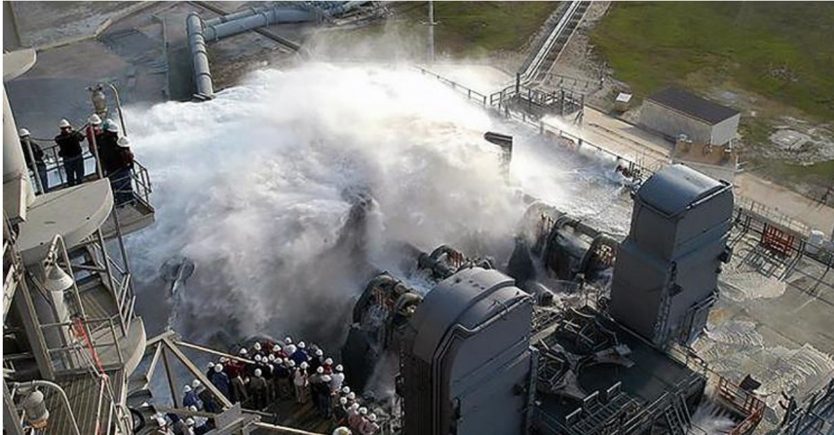
Figure 5 Kennedy Space Centre Launch Pad 39A water sound suppression system (NASA - https://www.nasa.gov/missions/shuttle/f_watertest.html )
