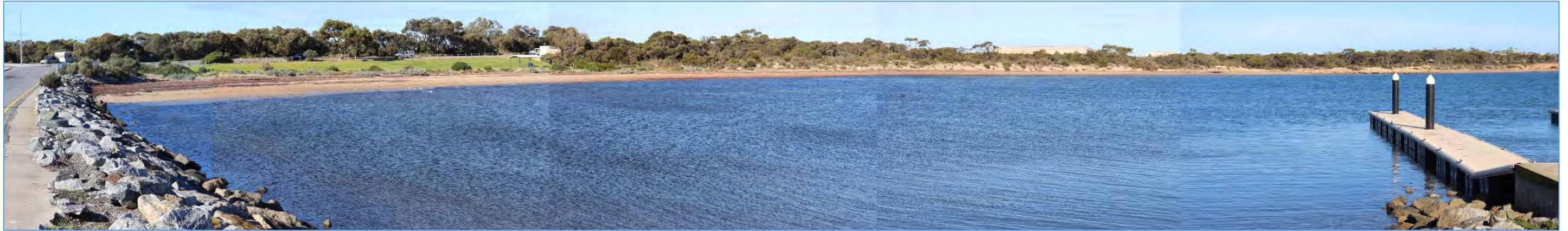
Image 1: Panoramic view at Billy Lights Point and ex-BHP sand storage shed.
