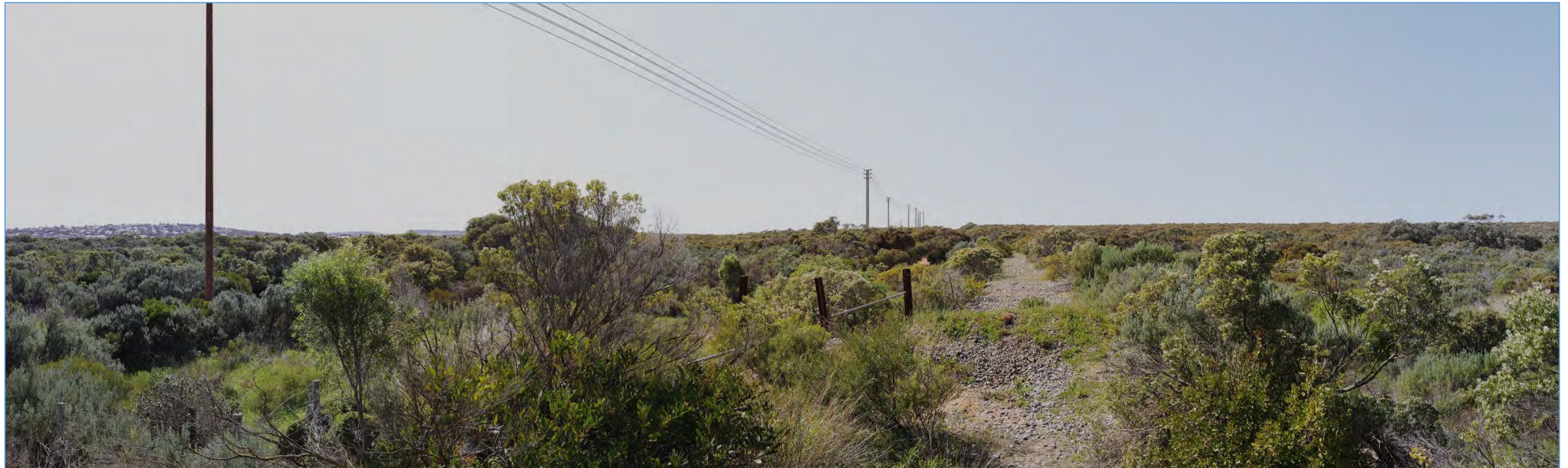
Image 18: SR 04 – Photomontage view of The Project powerlines from Greyhound Road, view east
