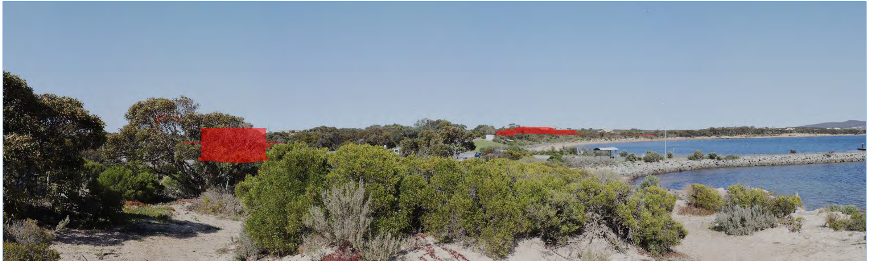
Image 19: SRL01 - View southwest from Billy Lights Point Reserve – x-ray image indicating The Project's desalination plant and intake pumping station
