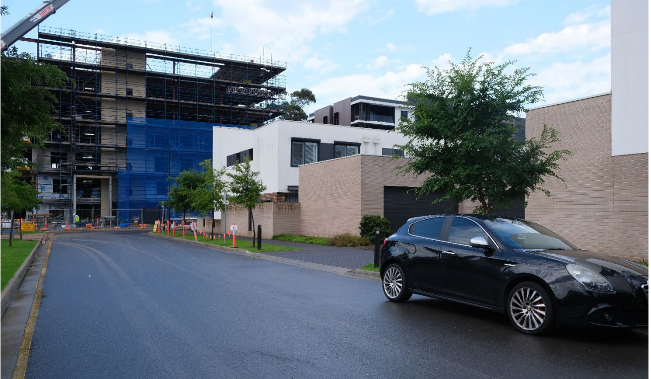
Figure 8 Banksia Street / terrace housing and apartments under construction
