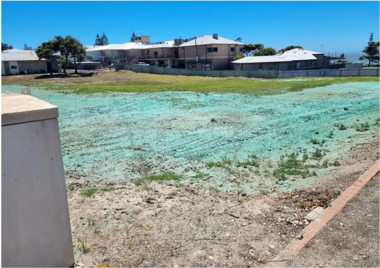
Figure 1: Southern Side of Site Looking North-East Across Area for New Road
