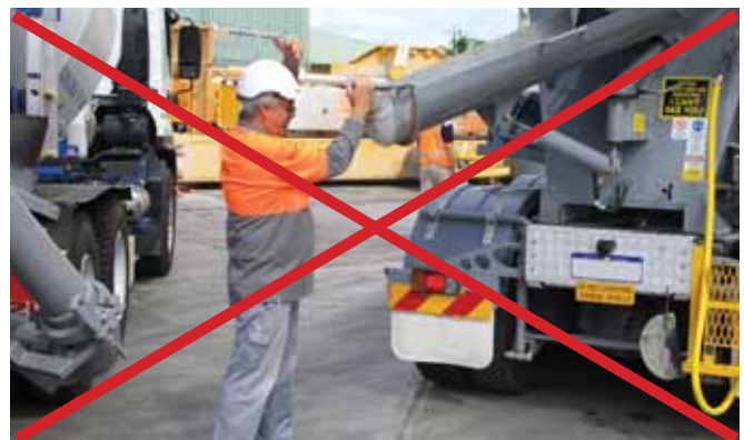
Unsafe spotter without appropriate PPE and position adjusting concrete chute while truck is reversing
