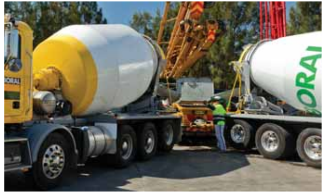
A truck spotter, in correct PPE, reversing a concrete agitator onto the concrete pump. Two trucks on the feed with over 600mm clearance.
