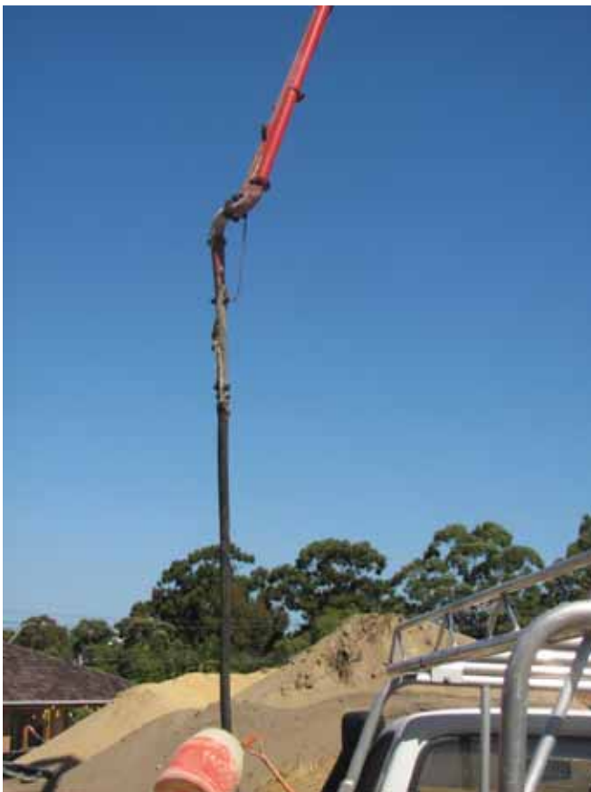
Delivery hose secured by safety chain
