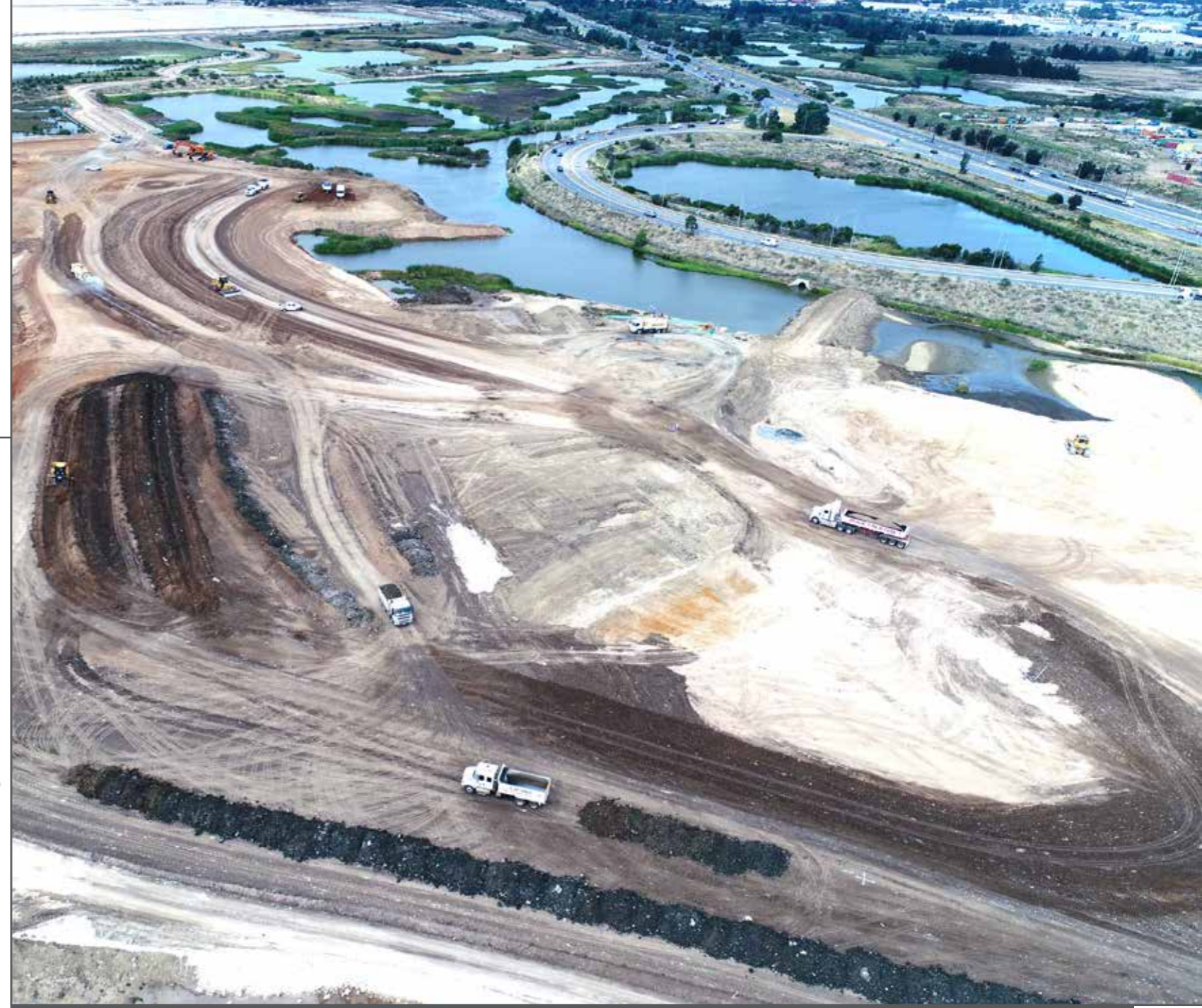
>> Current works in the Southern Interchange, along the Port River Expressway
