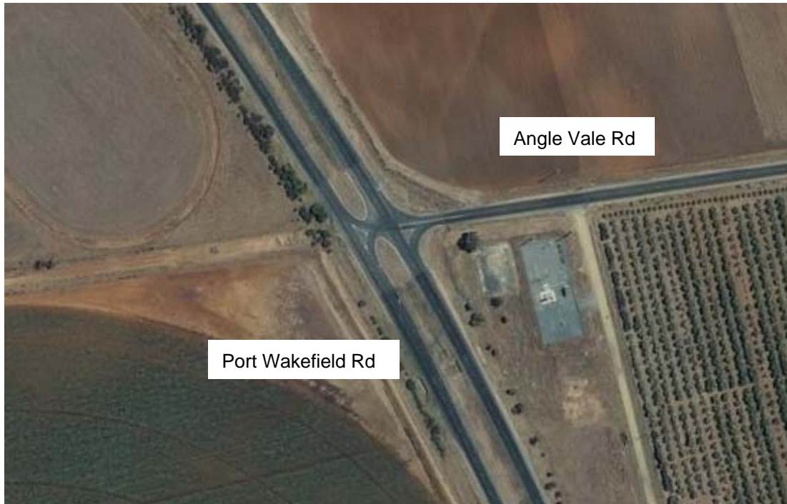
FIGURE 5.4 Existing intersection of Port Wakefield Road and Angle Vale Road
