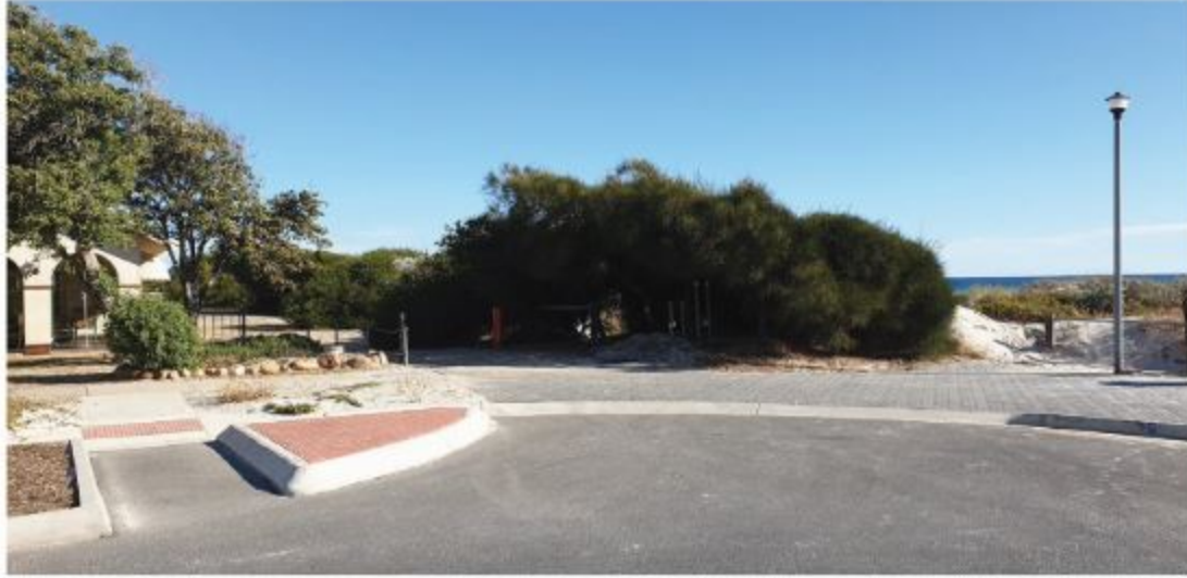
BEFORE - Third Avenue
