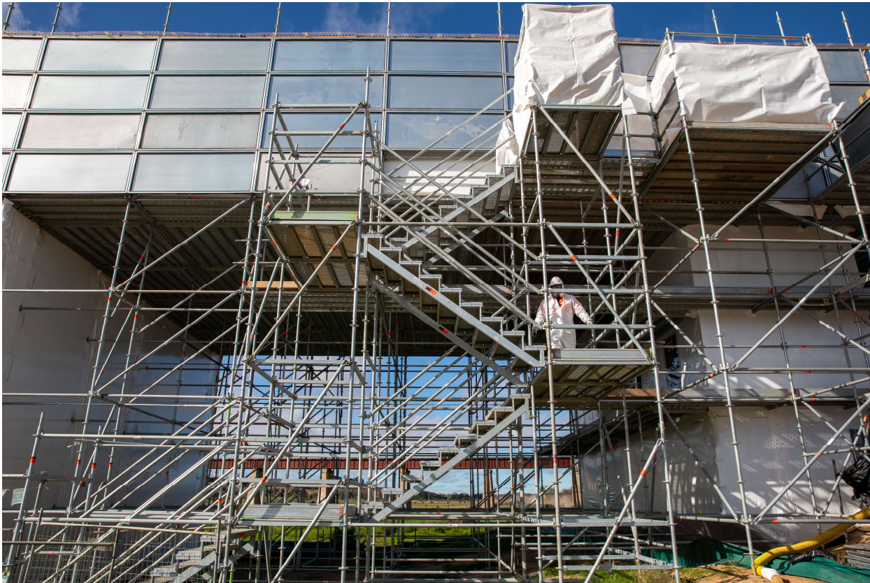
Image: Worker access through airlock system
