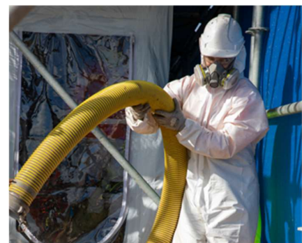
Image: Worker wearing Personal protection Equipment
