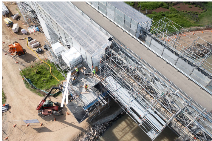
Image: Scaffolding and Encapsulation under construction
