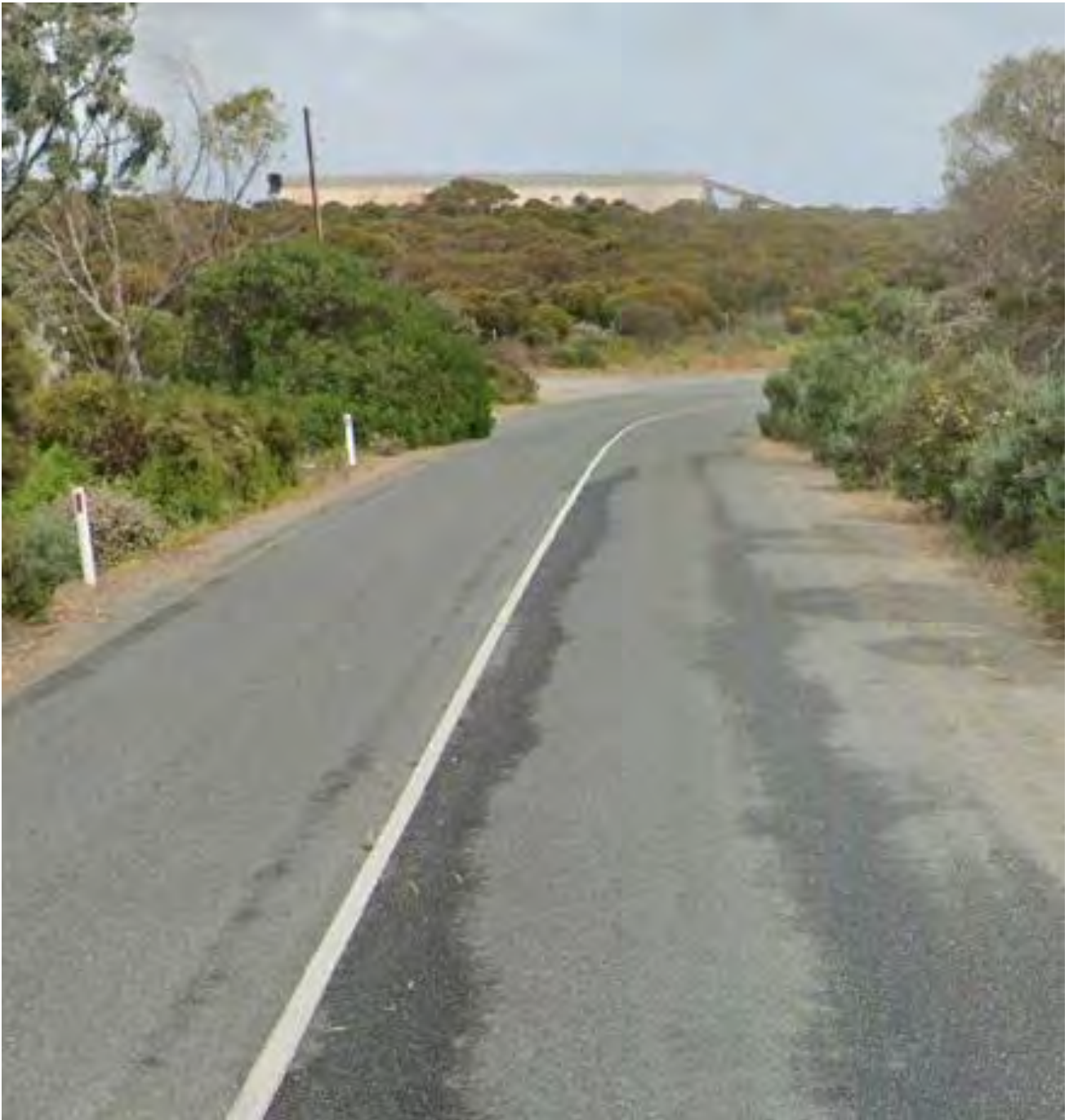
Figure 2.9 Restricted visibility of the WWTP access road junction
