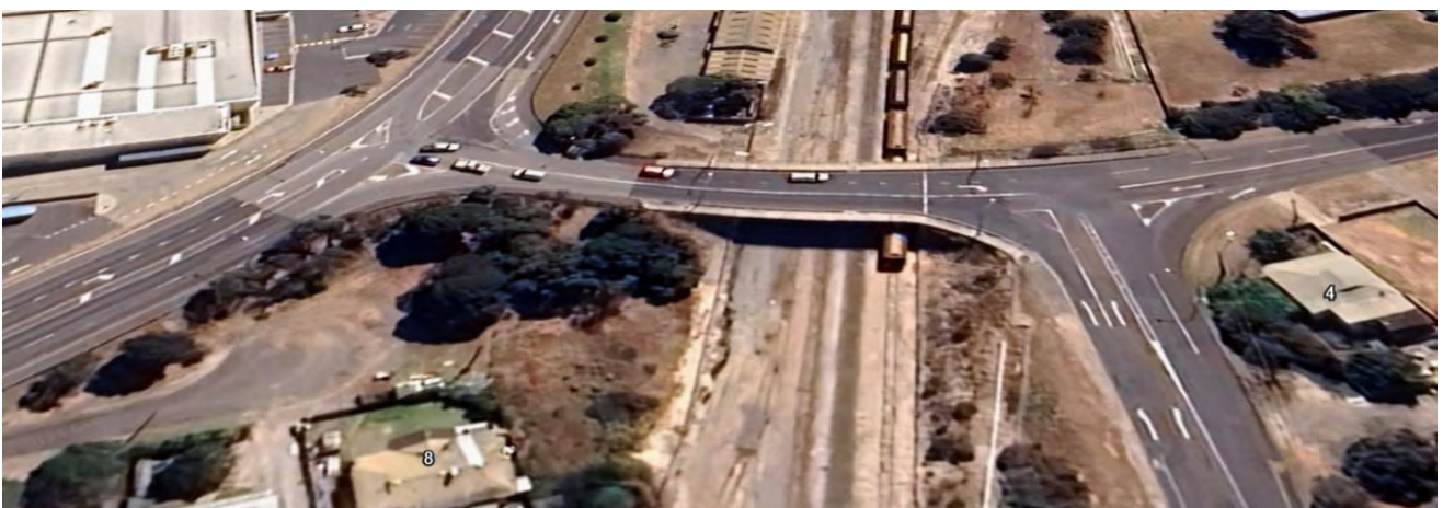
Figure 2.4 Junctions Dublin Street-Porter Street and Dublin Street -Luke Street
