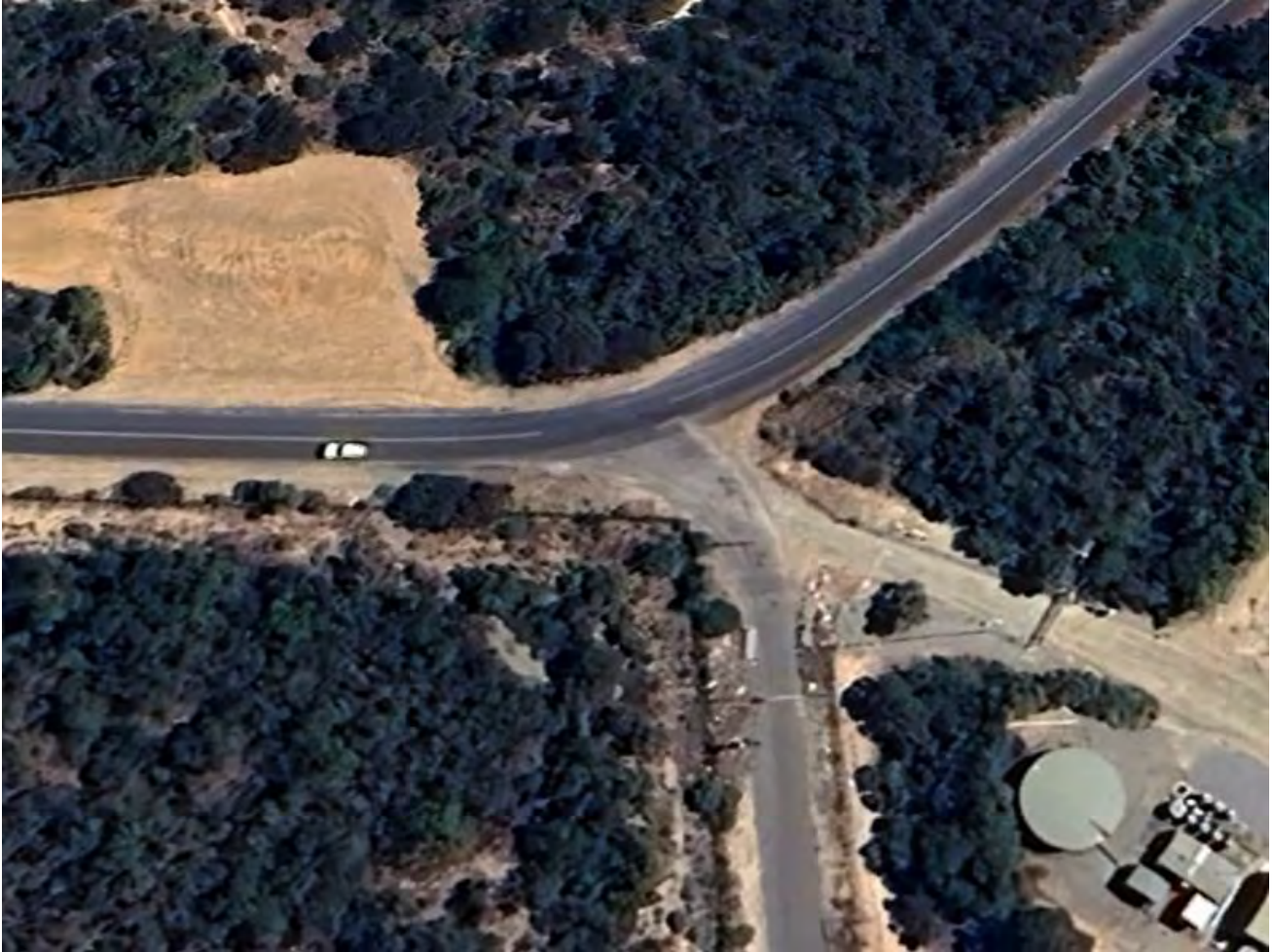
Figure 2.8 WWTP access – St Andrews Drive
