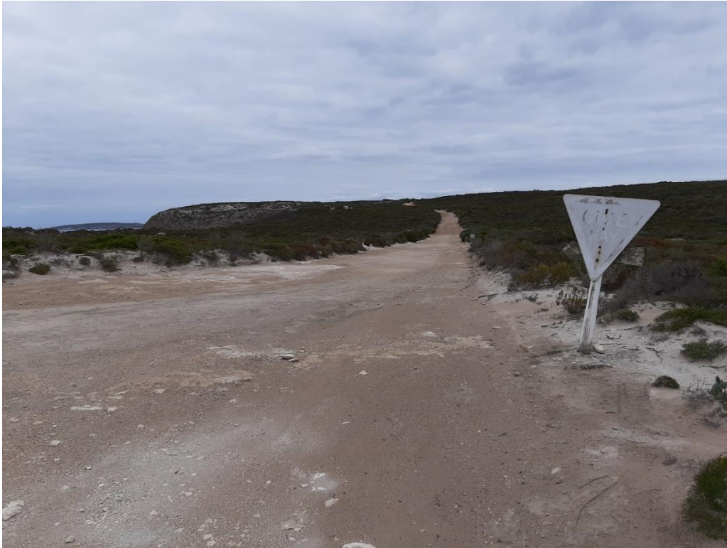
Figure 21 – Sink Hole Road Junction Looking Westerly, note faded “give way” sign (eastbound SISD is good > 106m). This intersection is currently in operational (Sink Hole Road is closed).
