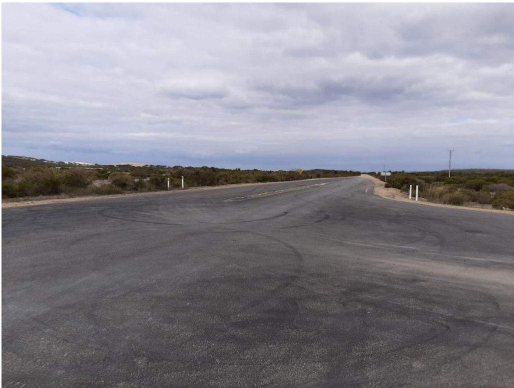
Figure 14 - Proper Bay Road / Fishery Bay Road (Looking South)
