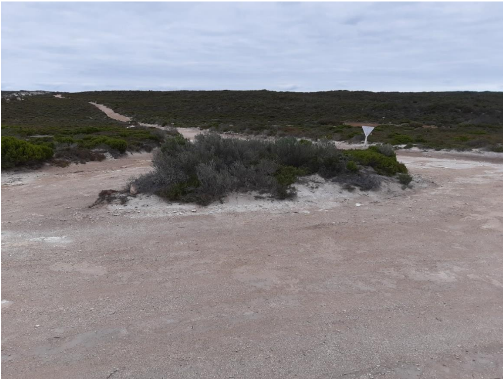
Figure 20 – Access Track Junction Layout “Sink Hole Road” (west end) – looking easterly (westbound SISD is good > 106m). This intersection is currently in operational (Sink Hole Road is closed).
