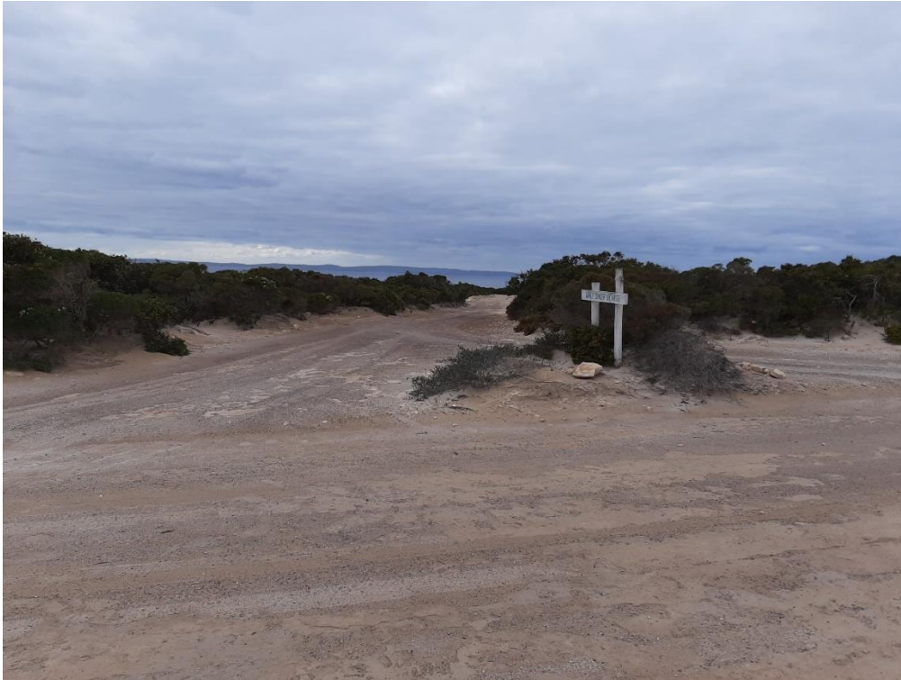
Figure 17 – Access Track Junction Seagull Layout “Whale Chaser Crevasse” (looking south). The junction with the minor access track Whale Chaser Crevasse provides reasonably good ASD (>55m) on approach to the major access track.
