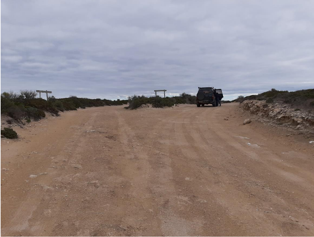
Figure 19 – Access Track Junction Layout “Mathew Flinders Lookout” (west end – looking westerly). This junction has a particularly poor intersecting angle
