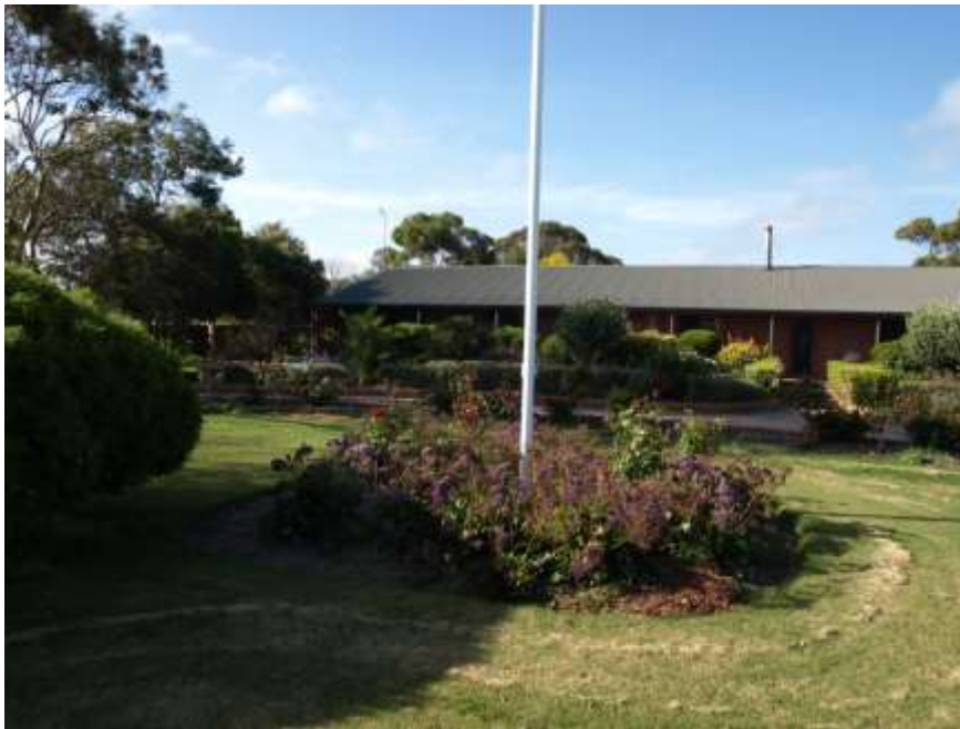
Photo 4 Residential property (6-8 Banfield Road) that is to be demolished.
