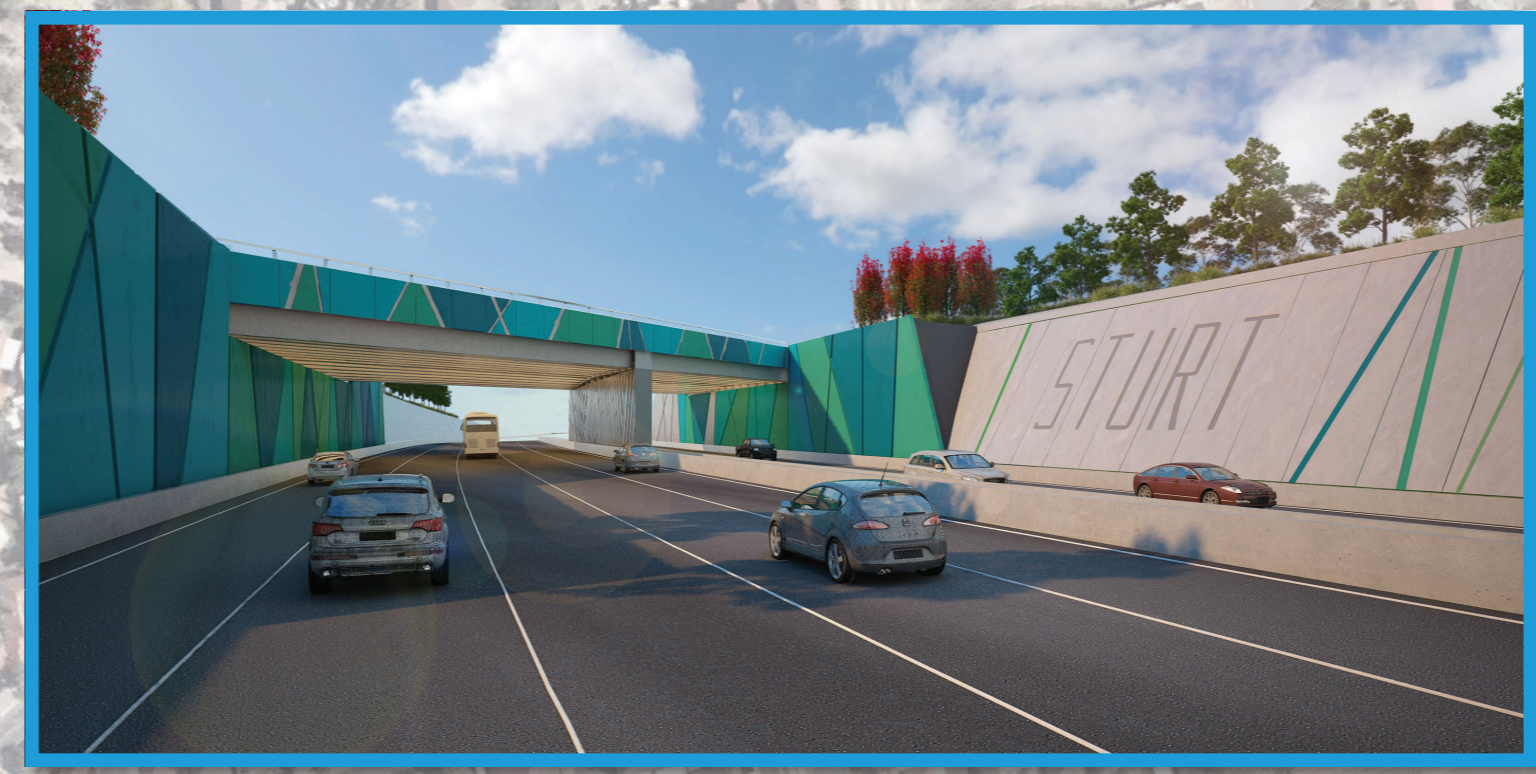
Artists impression of lowered motorway retaining walls with embossed road
