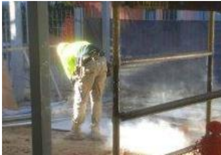
RCS produced while cutting cement fiber boards
