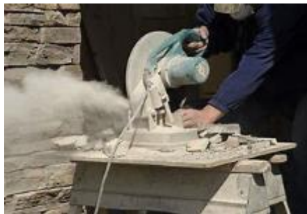
RCS being produced during cutting
