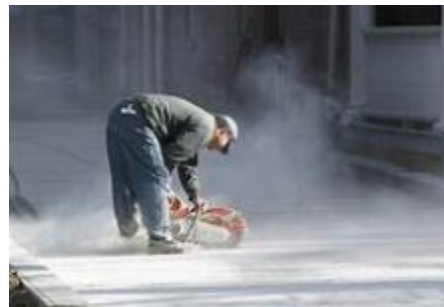
Using a quickcut is a common way by which RCS is created
