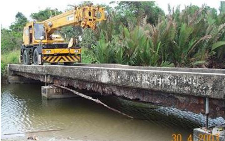
Figure 1: Girder corrosion grossly ignored over long period (PNG)
