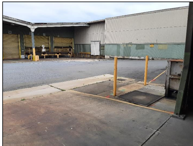
Photograph 3 – view of the interceptor adjacent the former wash bay
