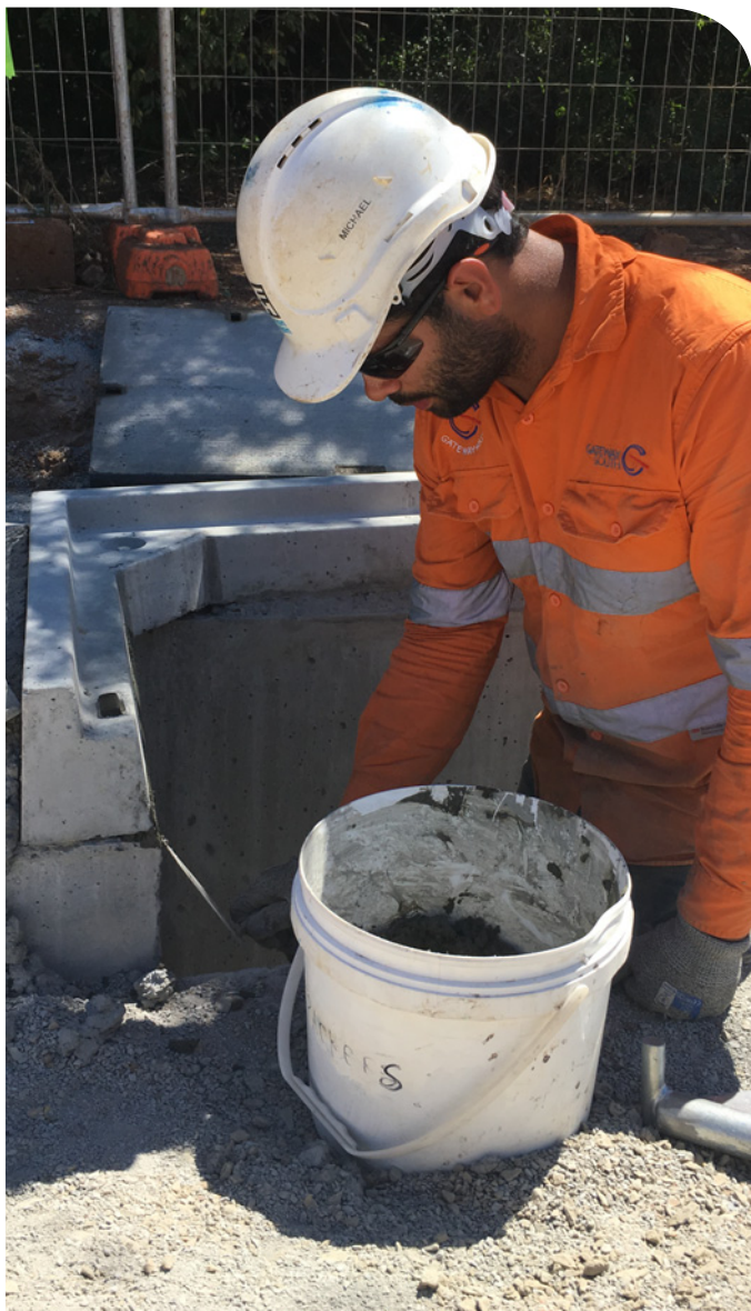
Michael Sumner recently obtained his Certificate 3 in Civil Construction whilst working on the Darlington Upgrade Project
