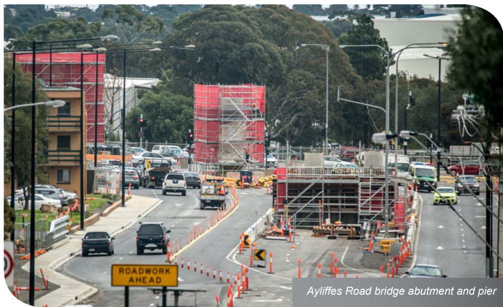
Temporary supports for the northern section of the Ayliffes Road bridge
