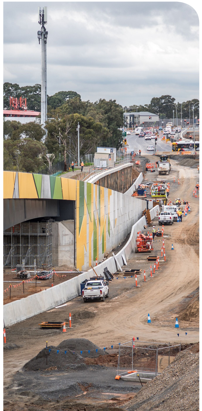
Northern abutment of the Main South Road bridge over the Southern Expressway onto surface roads
