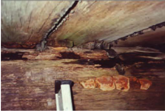
Figure 29: Fungal fruiting body and decay of girder
