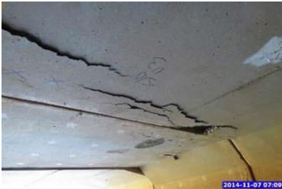
Figure 5: Delamination in culvert slab
