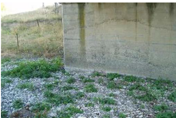
Figure 12: Cold joints in abutment wall
