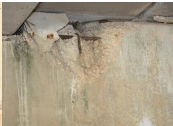
Figure 7: Spalling to front face of headstock
