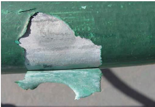
Figure 34: Failure of paint system over galvanising
