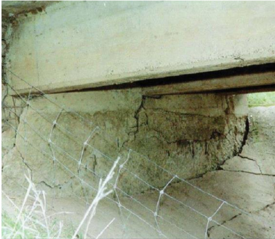
Figure 2: Disintegration of concrete
