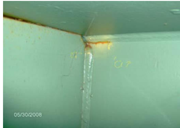
Figure 23: Cracking in welds
