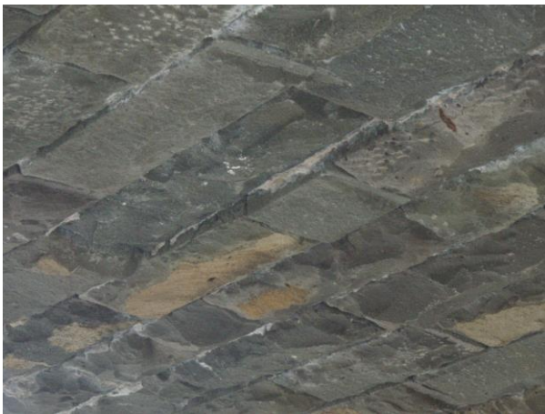
Figure 28: Dropping of arch masonry block
