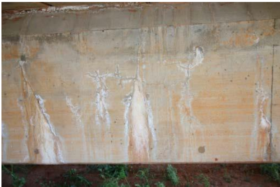
Figure 13: Efflorescence evident on concrete headstock
