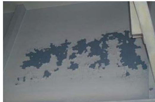
Figure 36: Flaking of paint system
