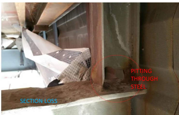
Figure 19: Section Loss and Pitting Through Steel
