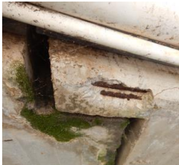
Figure 4: Corrosion of reinforcement in concrete
