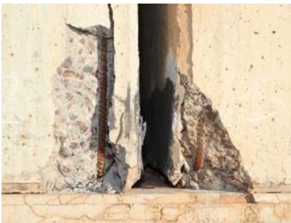
Figure 6: Spalling of concrete at ends of deck units
