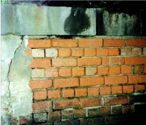
Figure 27: Loss of mortar
