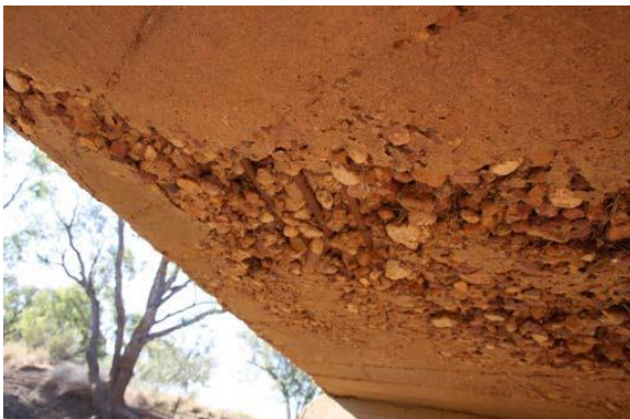
Figure 15: Concrete honeycombing
