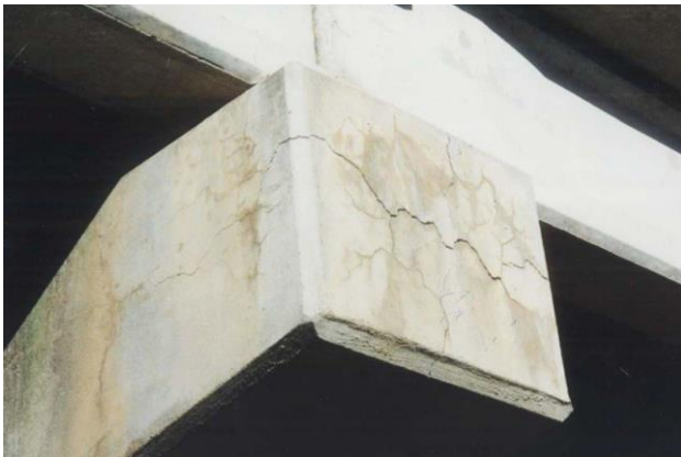
Figure 10: Concrete affected by alkali aggregate reaction (AAR)
