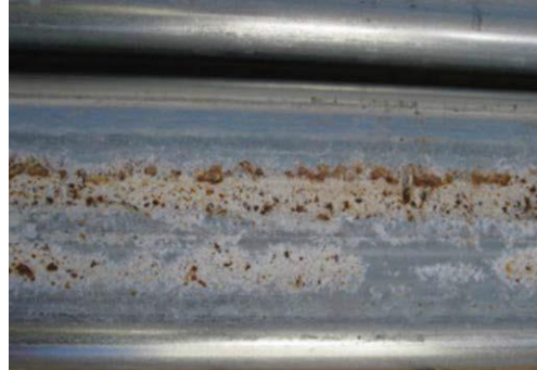
Figure 33: White deposit on zinc metal spray
