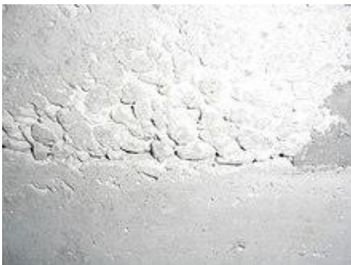
Figure 11: Concrete segregation
