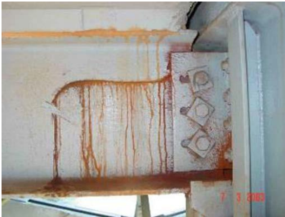
Figure 22: Fatigue cracking in web
