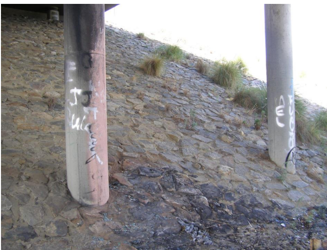
Figure 17: Fire damage to concrete column
