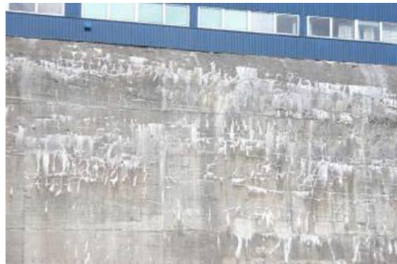
Figure 14: Discharge through cracks in concrete surface
