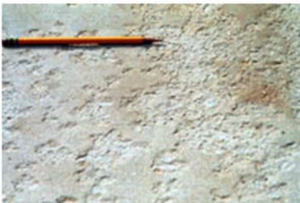
Figure 1: Concrete scaling
