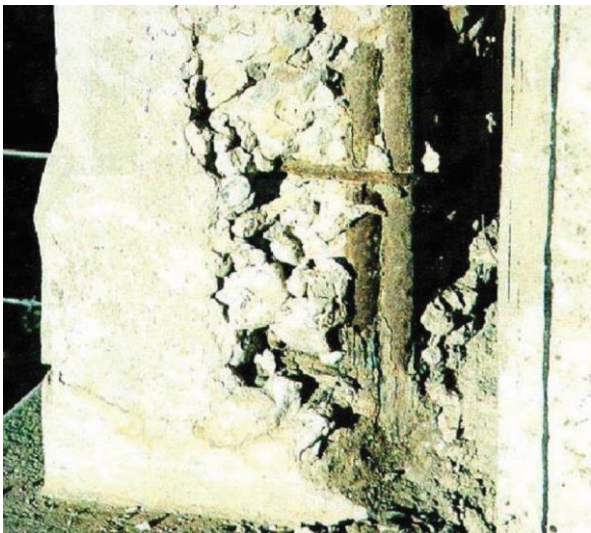
Figure 3: Corrosion of reinforcement in concrete
