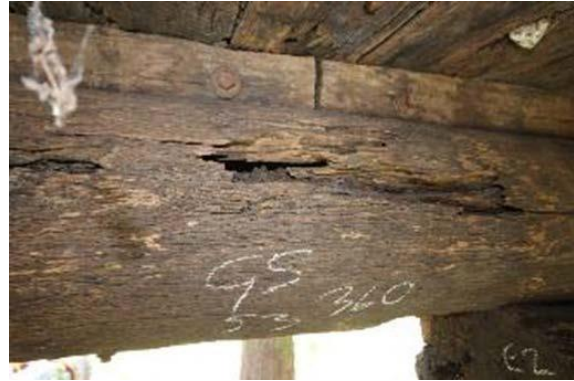
Figure 30: Decay pocket in girder
