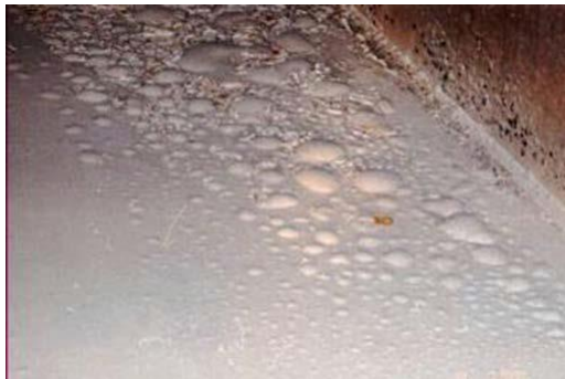
Figure 35: Blistering of paint system
