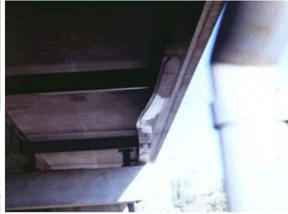
Figure 21: Impact damage to steel beam
