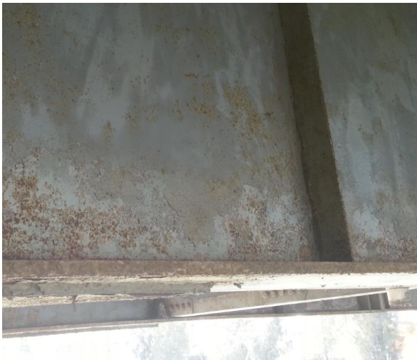
Figure 18: Light corrosion on steel work and loss of protective coating
