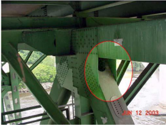
Figure 20: Buckling of gusset plate
