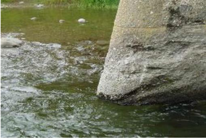
Figure 16: Erosion of concrete due to water wash
