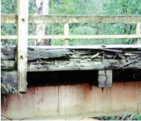
Figure 31: Termite attack
