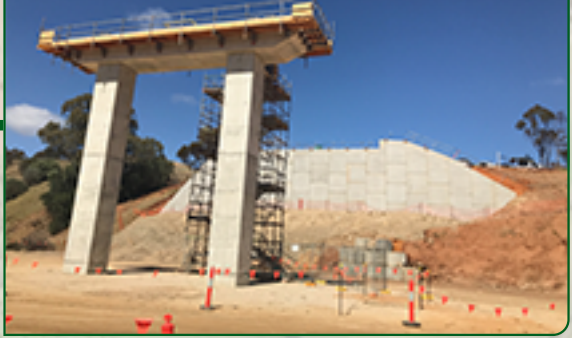
Construction of the bridge piers - December 2019
