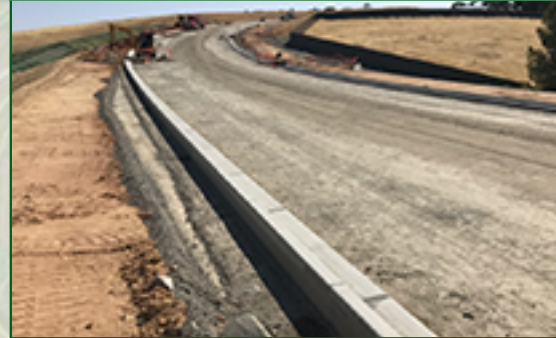
Kerbing the new link between Potts Road and Gawler-One Tree Hill Road - January 2020
