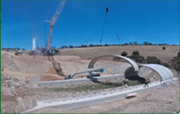
Construction of the Bebo Arch structure - December 2019
