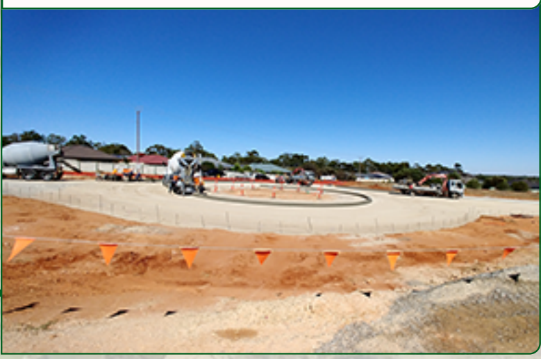
Construction of the Potts Road roundabout - January 2020
