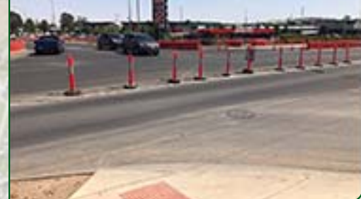
Road widening and asphalt works on the Tulloch Road Intersection Upgrade Project - January 2020
