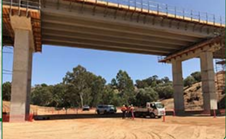
Looking underneath the bridge deck - January 2020
