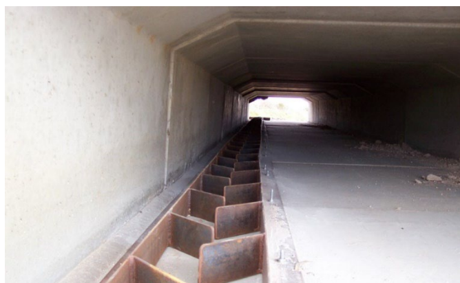
Figure A-3 Fish ladder in culvert traversing Margaret Creek along the Oodnadatta Track
