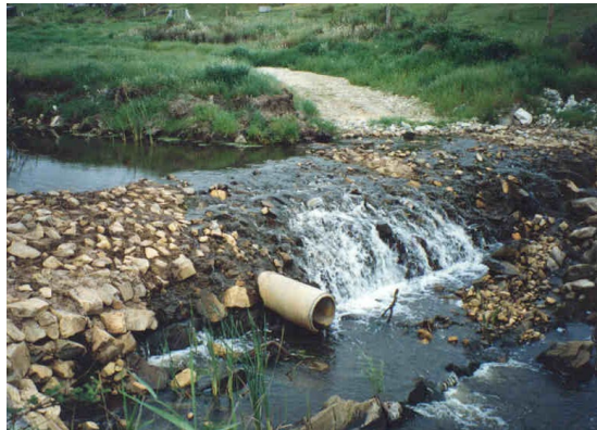
Figure A-1 Roughened surface provides a fish ladder in Tookyerta Creek
