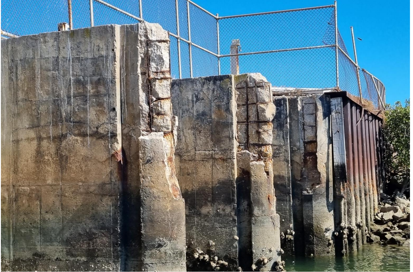
Figure 10: Existing tidal gates
