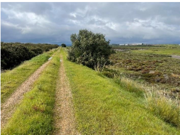
Figure 32: Image of existing levee (view to the east).
