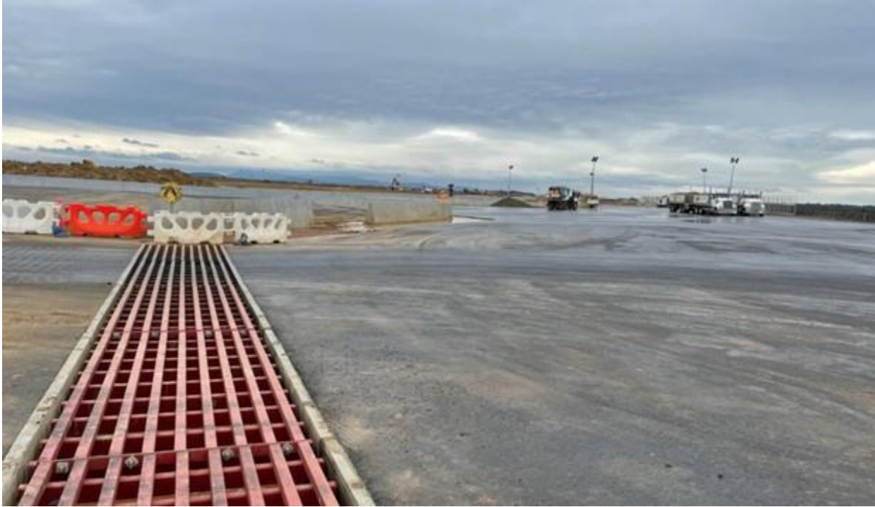
Figure 13: Example of a spoil receipt and handling area
