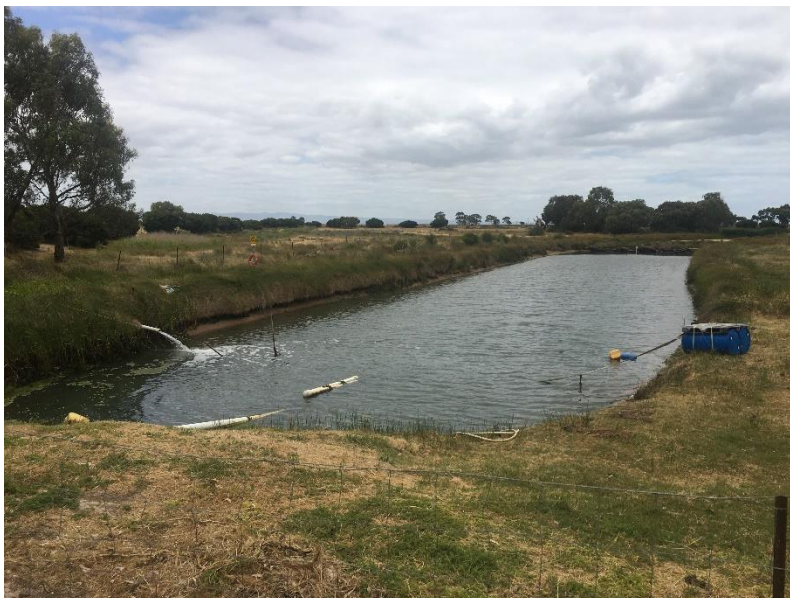
Photograph 13. Detention basin behind shed on adjacent property to the west. 14.12.2022
