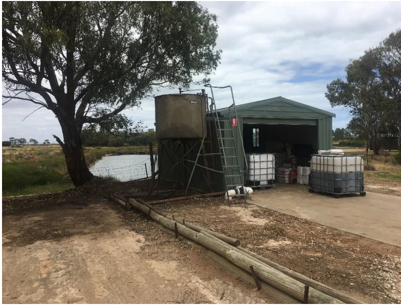
Photograph 11. Pump shed, diesel AST and IBCs on adjacent property to the west. 14.12.2022
