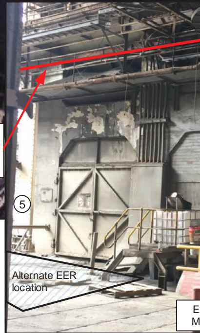
New cable ladder to extend existing Sinter North MCC feeder cables to new Pre-Treatment MCC
