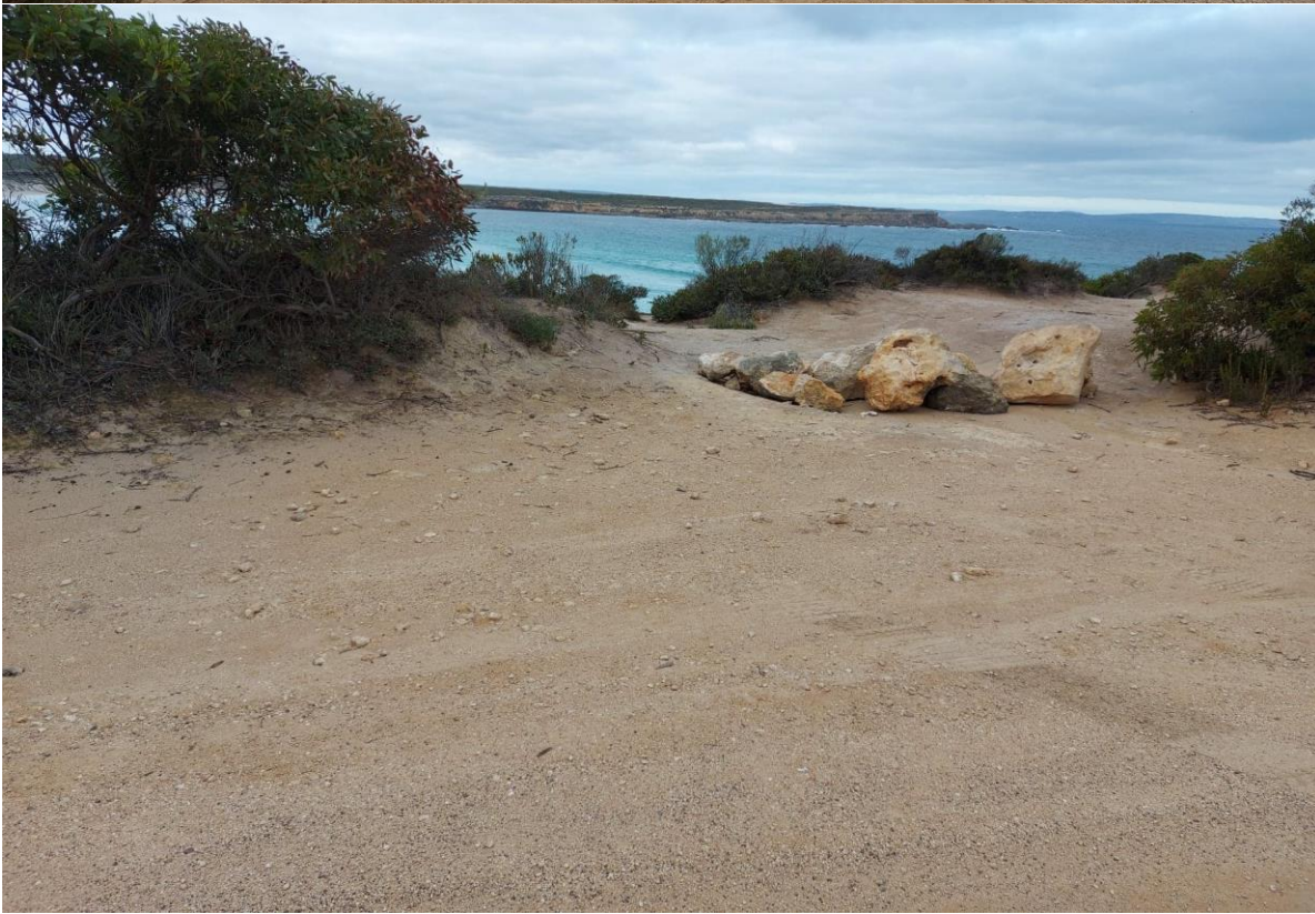
Figures 1 and 2: The road in some places skirts less than 10 metres from highly unstable limestone cliff edges.
