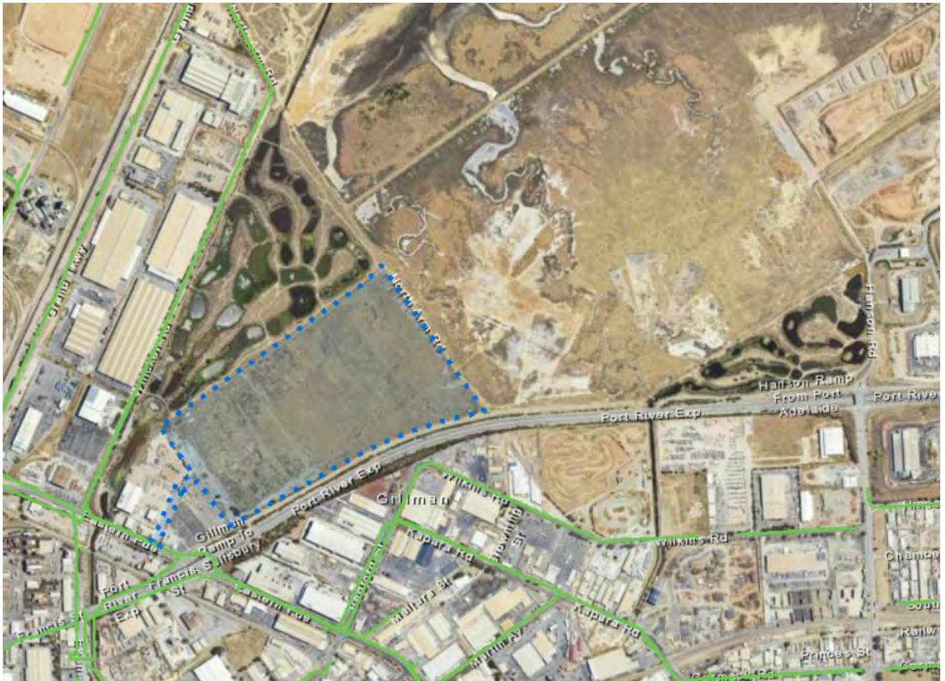
Figure 17. SA Power Networks Subtransmission and High Voltage Overhead Line (Green) (Source: SAPPA, 23 February 2024)
