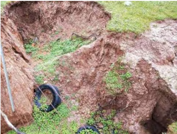
Figure 7.3 Active erosion was recorded at several locations within the River Red Gum creekline
