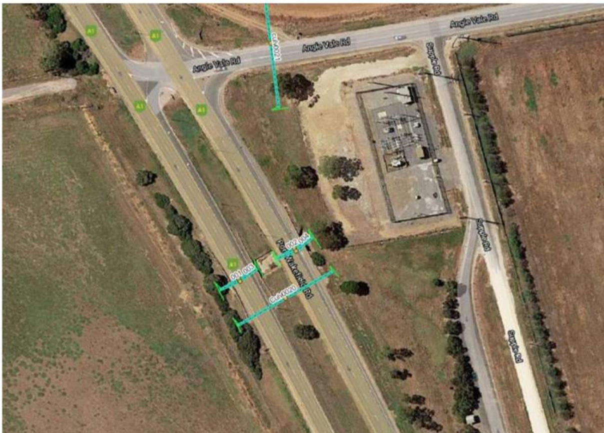
Figure 10: Port Wakefield Road Culverts
