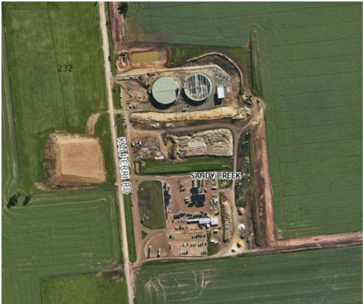
Figure 3 – Aerial image of the subject site showing construction of approved tanks underway
