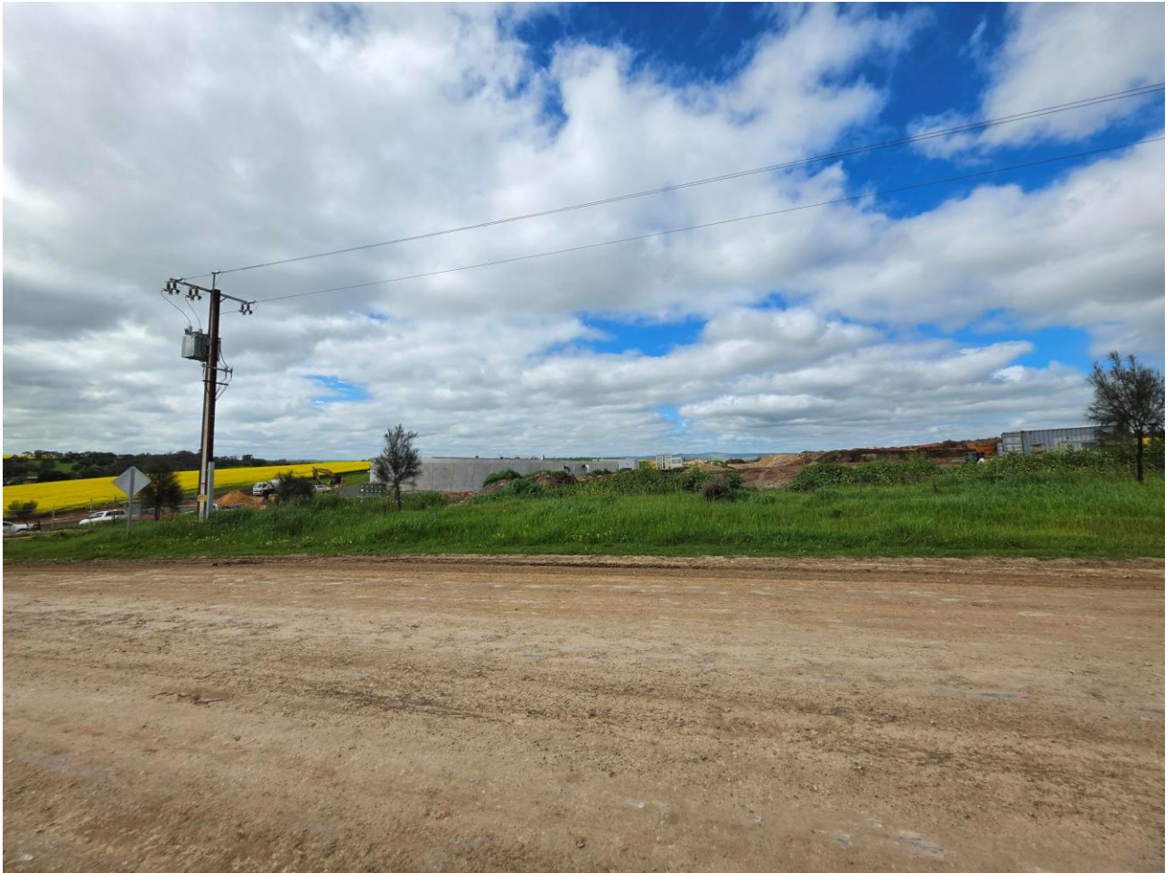
Figure 5 – Photograph looking east at the subject site and existing tanks under construction
