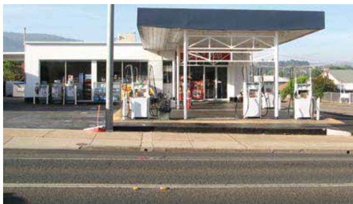
Picture shows an undersized canopy with fuel pumps outside the canopy dripline
