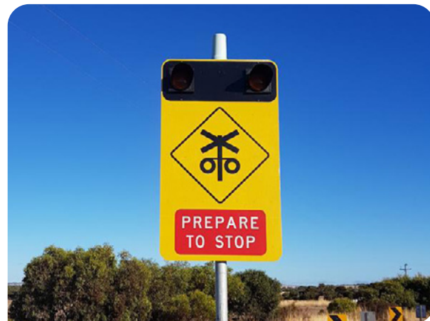
Figure 10. Example of an Active Advance Warning Sign
