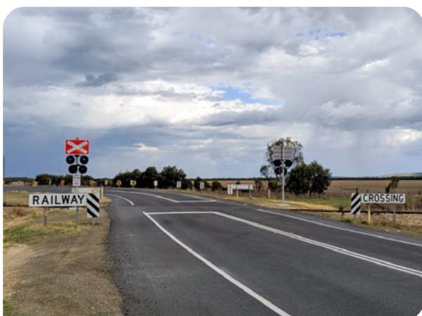
Figure 2. Example of an active level crossing – primary flashing lights (no boom gates)
