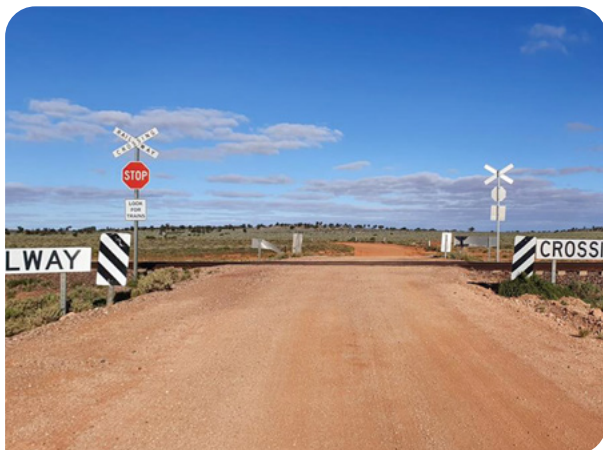
Figure 5. Example of a passive level crossing – Stop signs
