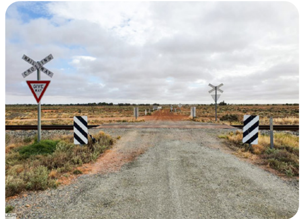
Figure 4. Example of a passive level crossing – Give Way signs
