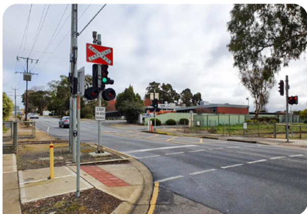
Figure 8. Example of a pedestrian actuated (push button) crossing at a level crossing
