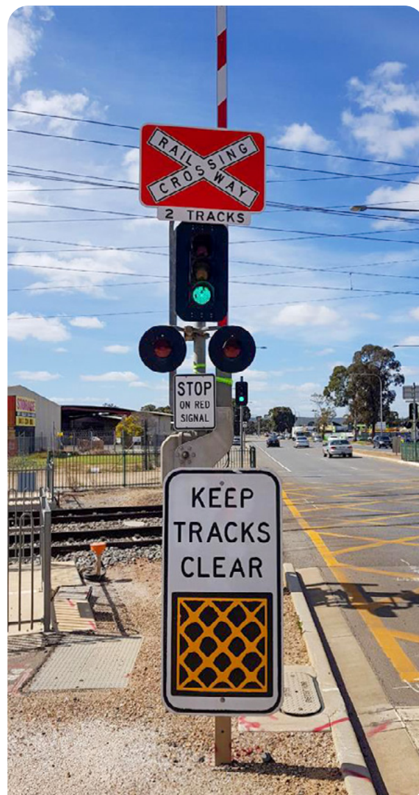
Figure 9. Example of a traffic signals secondary control with Queue Relocation Logic
