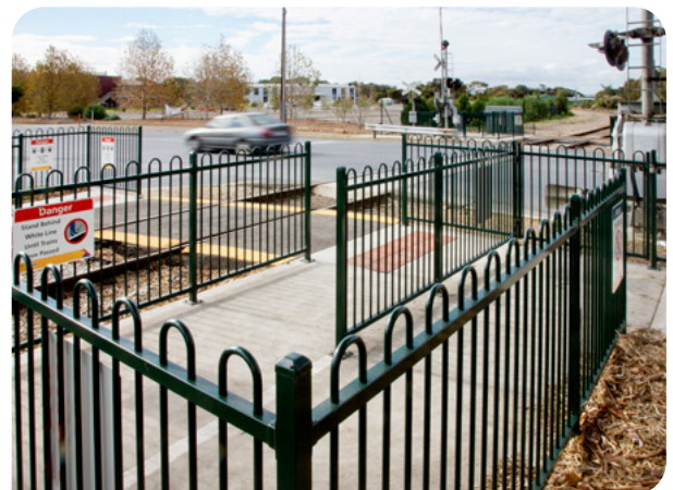
Figure 6. Example of a passive adjacent active road level crossing (pedestrian maze)
