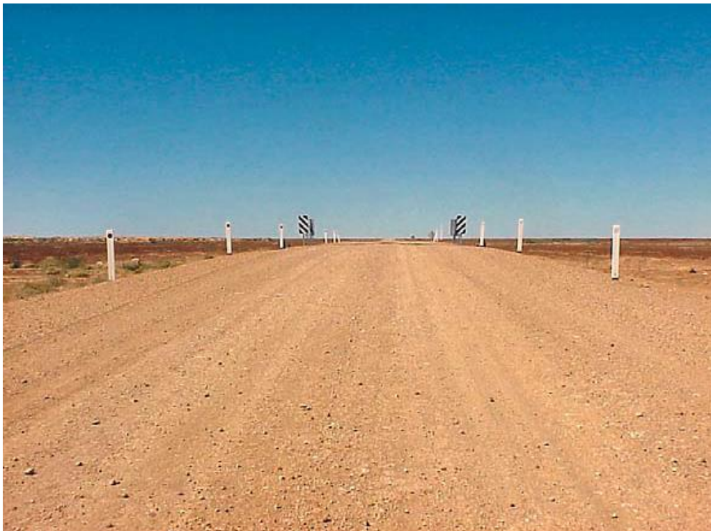
Photo 7 – Correct guide post installation at a grid
