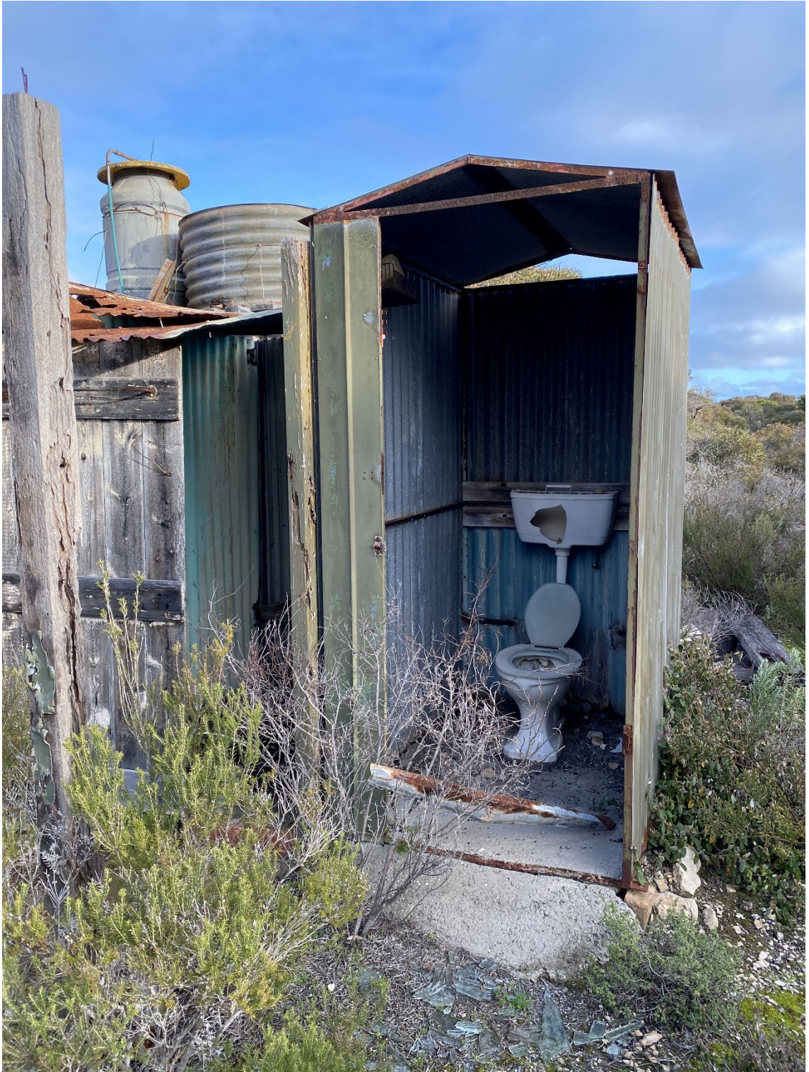
Photograph 3.20: Example of existing infrastructure at end of life.
