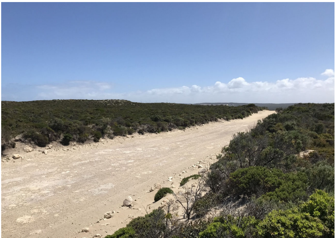
Photograph 3.22: Example of existing access roadway conditions.
