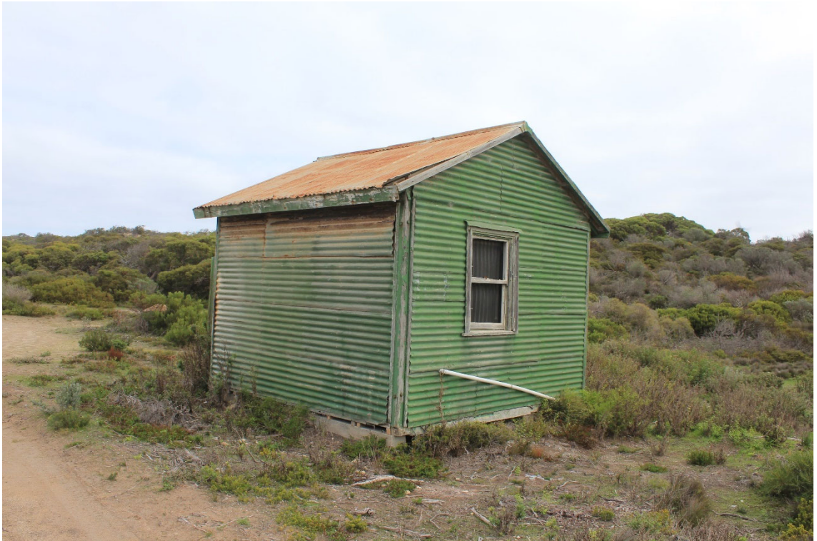
Photograph 3.11: Example of existing toilet infrastructure.
