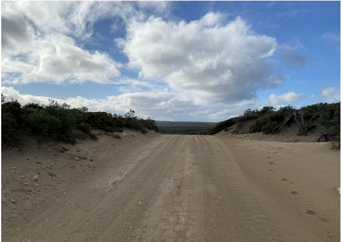
Photograph 3.23: Example of existing access roadway conditions.
