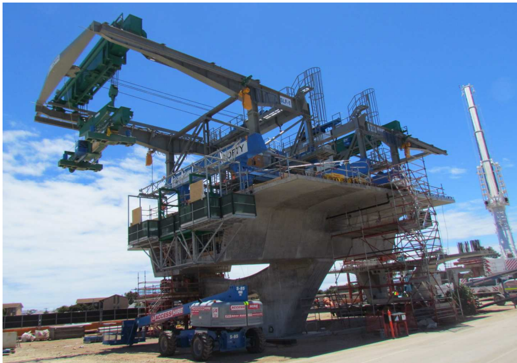
Segment Lifter on South Road, Regency Park
