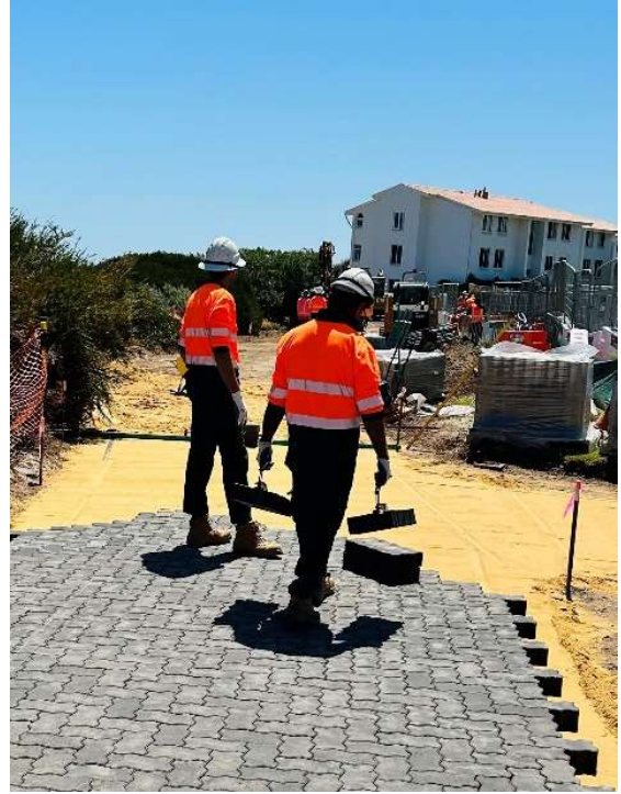
Mirani Court beach access paver installation
