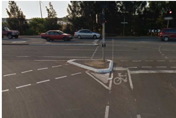
Figure 3: Lack of pedestrian ramps
