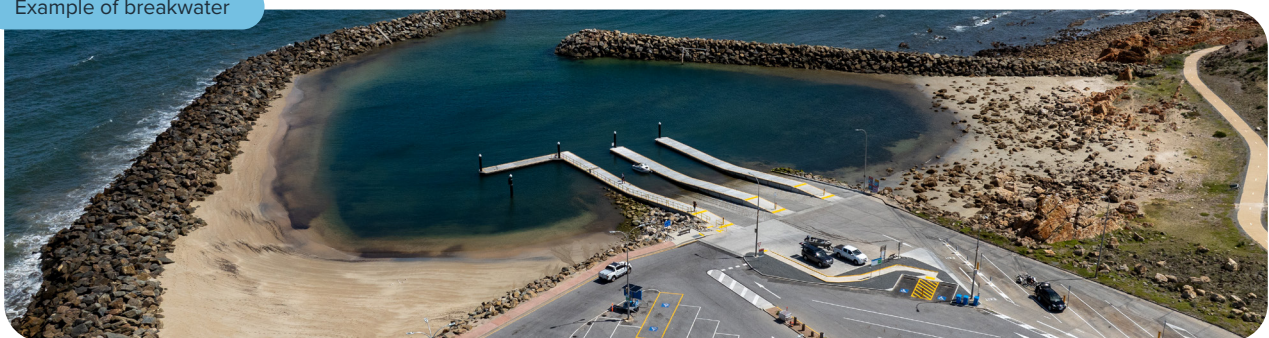
Figure 19: O'Sullivan's Beach breakwater
