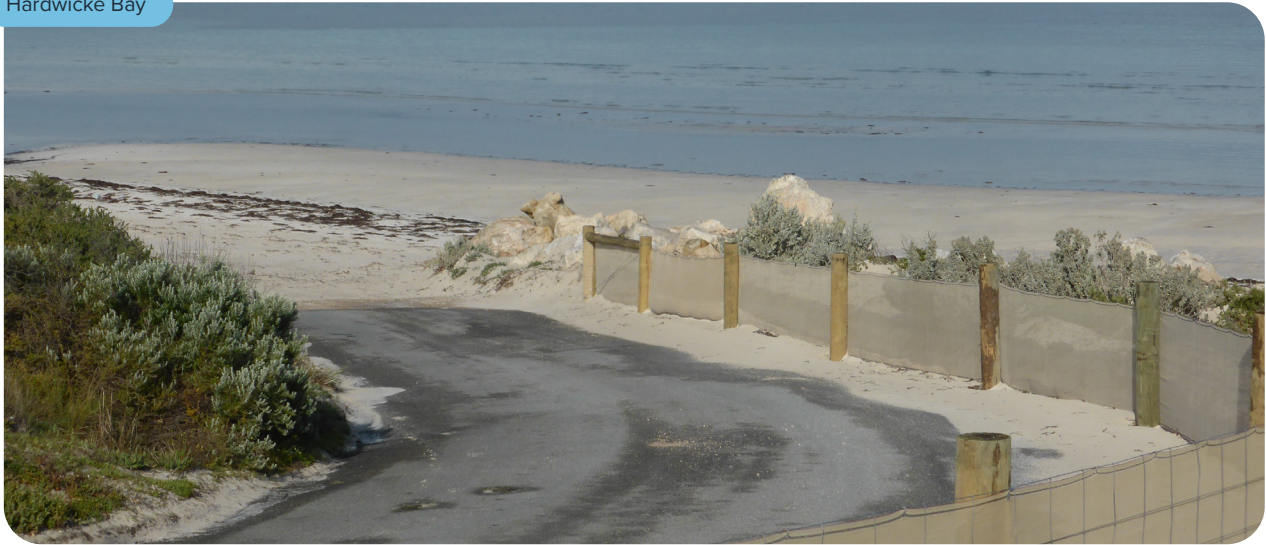
Figure 2: Service Level 1 launch facility at Hardwicke Bay
