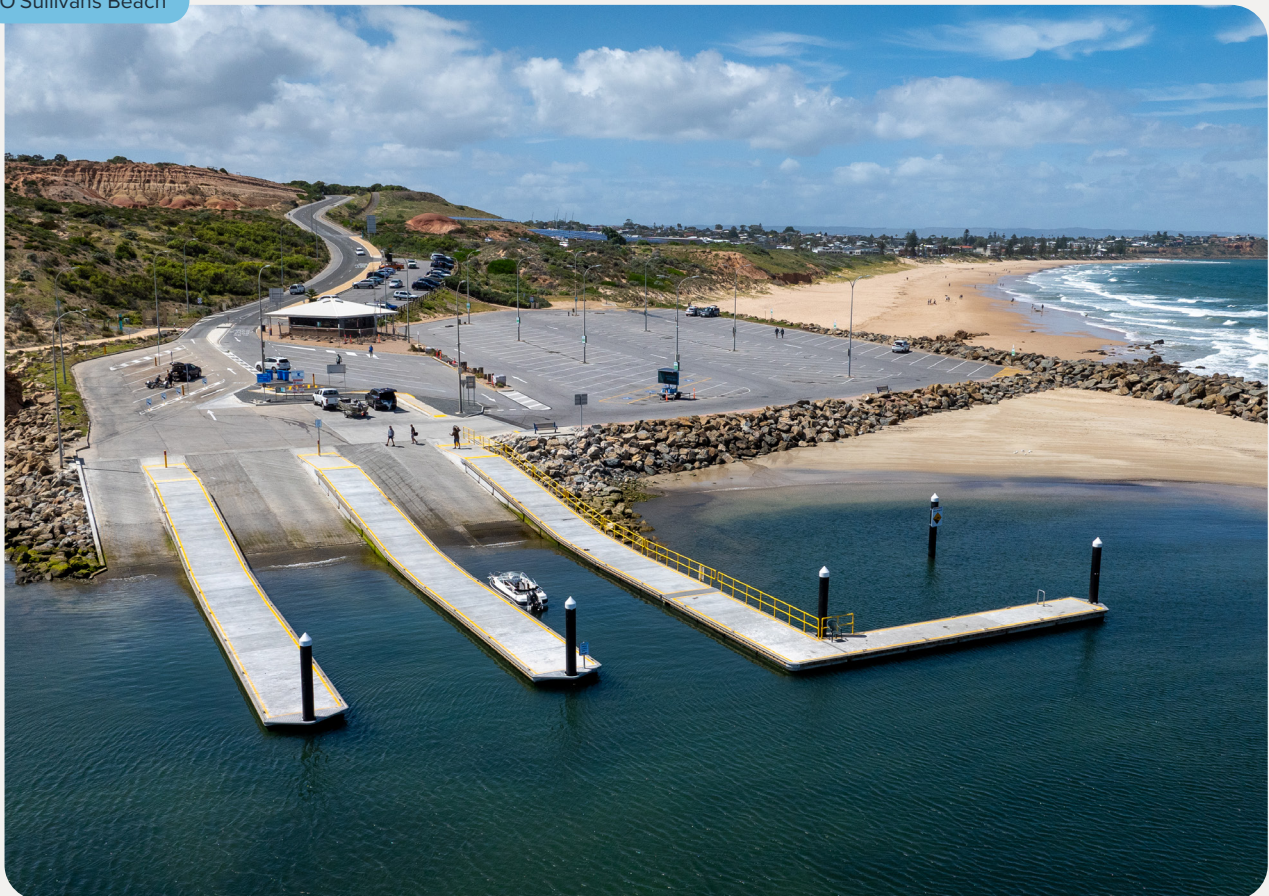
Figure 17: a boat launching facility at O'Sullivan's Beach
