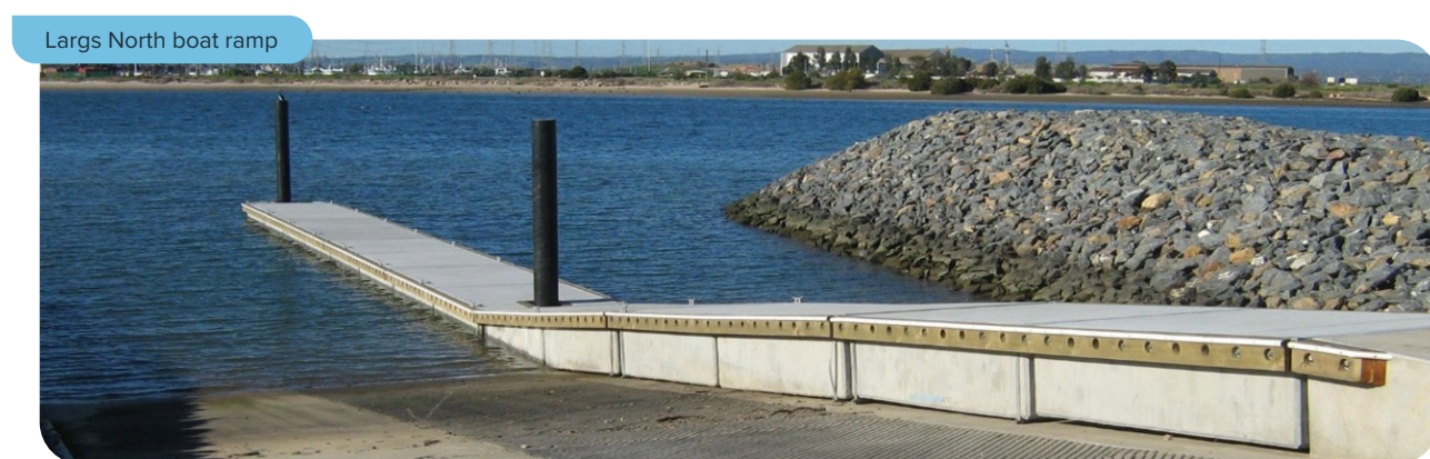
Figure 8: Boat ramp at Largs North
