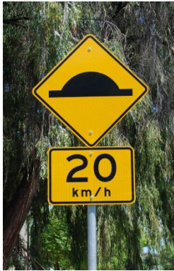
Figure 2.1 Good sign installation practice (no overlap)
