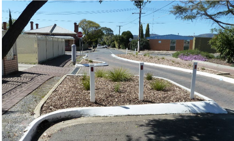
Figure 10.27 Example of drainage treatment at driveway entry
