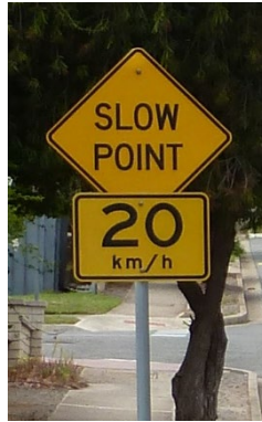
Figure 2.2 Poor sign installation practice (signs overlap)
