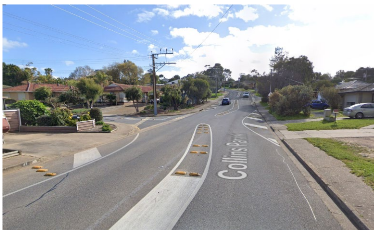
Figure 10.36 Modified T-intersection without change in priority (Collins Parade / Susan Road, Hackham) (Image from GoogleMaps "Street View")
