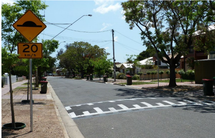
Figure 10.9 Watt's profile hump
