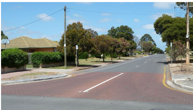
Figure 10.3 Contrasting pavement on approach to an intersection
