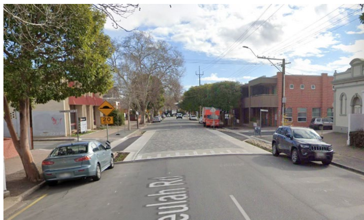
Figure 10.7 Example of raised pavement at a T-intersection extending into approaches on two legs (Beulah Road, Norwood) (Image from GoogleMaps "Street View")
