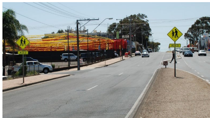
Figure 2.4 Duplicated pedestrian warning signs
