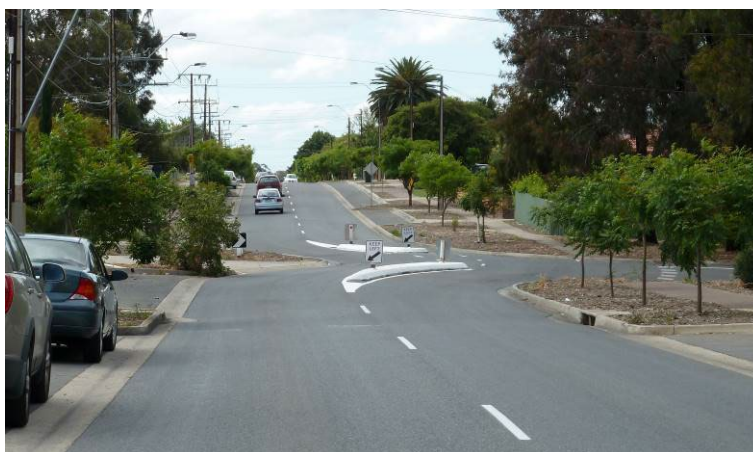
Figure 10.34 Modified T-intersection without change in priority (Valiant Rd / Southern Tce, Holden Hill)
