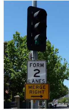
Figure 2.3 Poor installation practice (signs overlap, incorrect use and installation)
