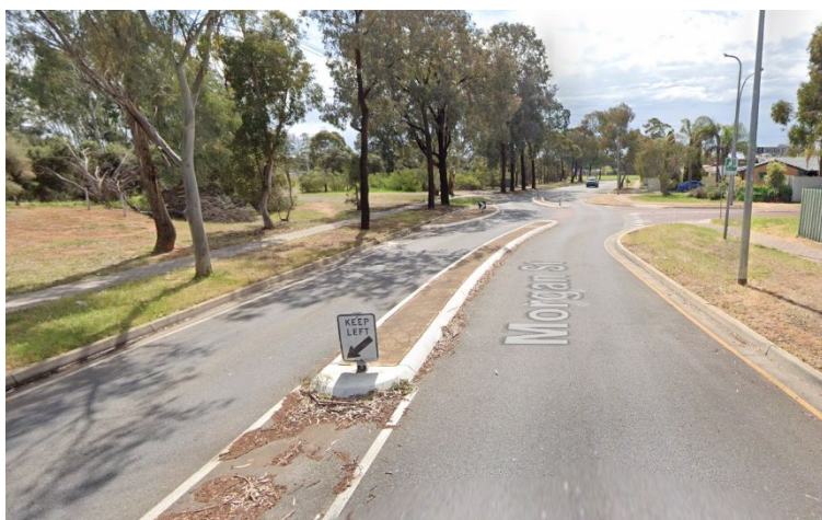
Figure 10.35 Modified T-intersection without change in priority (Morgan St / Watkin St, Parafield Gardens) (Image from GoogleMaps "Street View")
