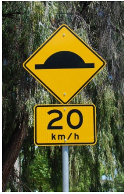
Figure 2.1 Good sign installation practice (no overlap)
