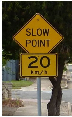
Figure 2.2 Poor sign installation practice (signs overlap)
