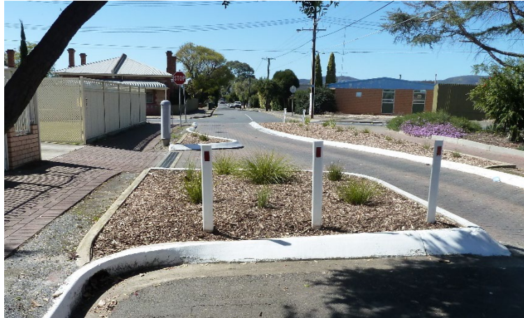
Figure 10.27 Example of drainage treatment at driveway entry
