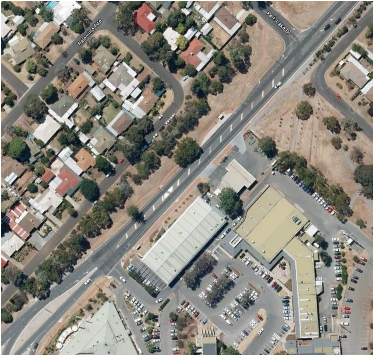
Figure 7.30: Golden Grove Road - Park Lake Drive to Grenfell Road (east)
