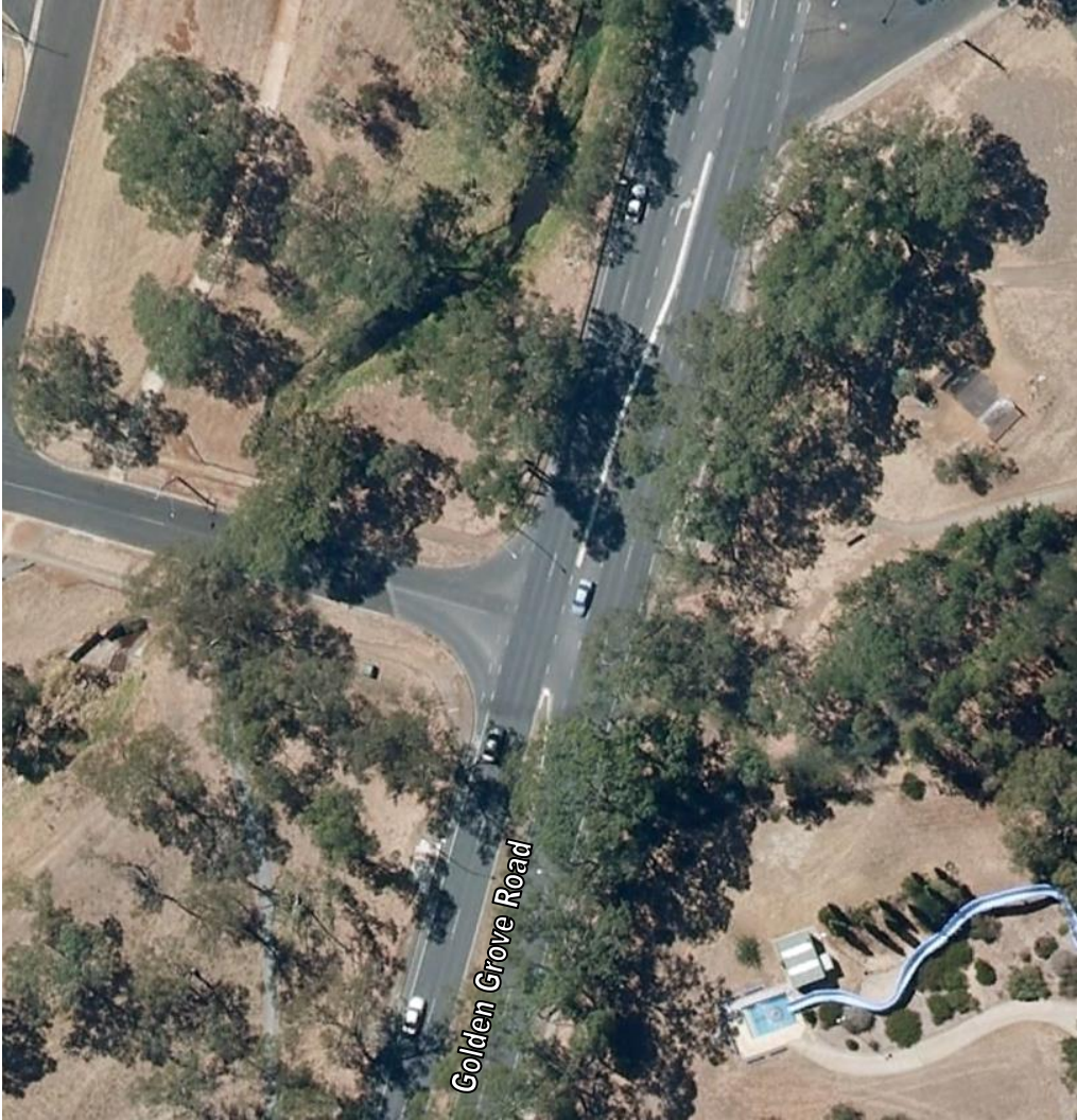
Figure 7.21: Golden Grove Rd / Oratanga Road Intersection
