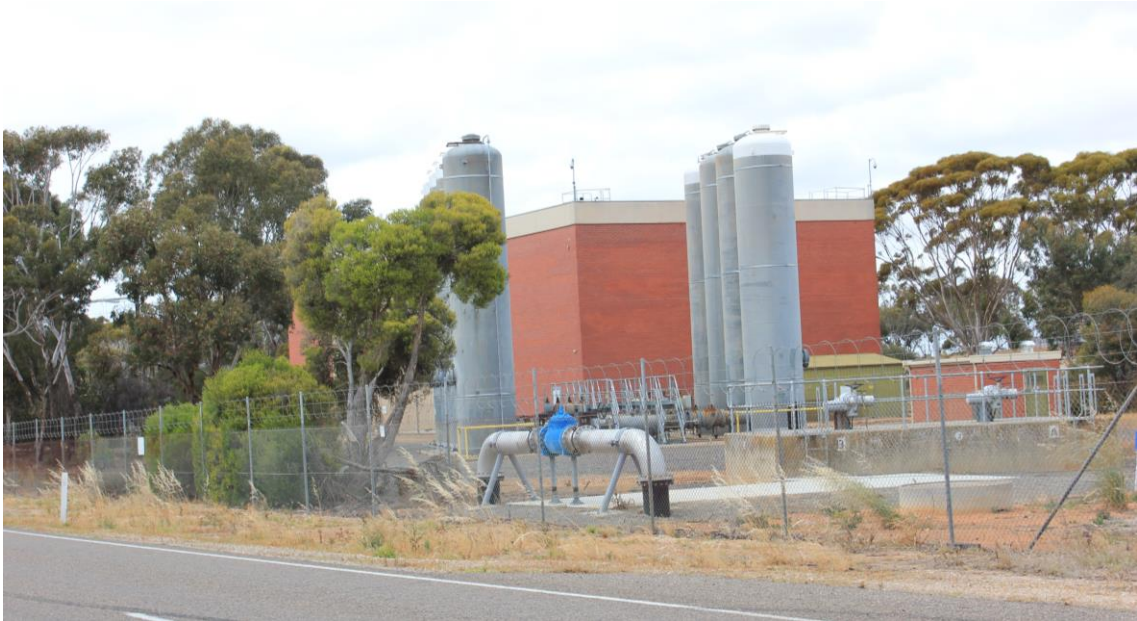
Figure 8: View of the SA Water pumping station along Monarto Road
