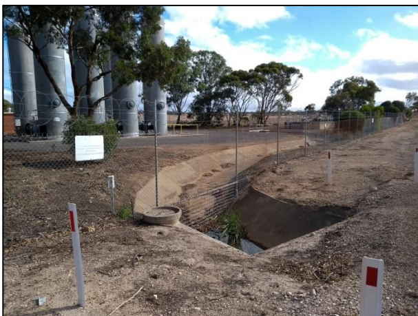
Figure 5 Drainage swale culvert
