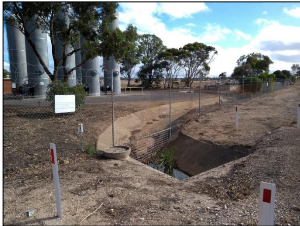
Figure 3 Drainage swale culvert
