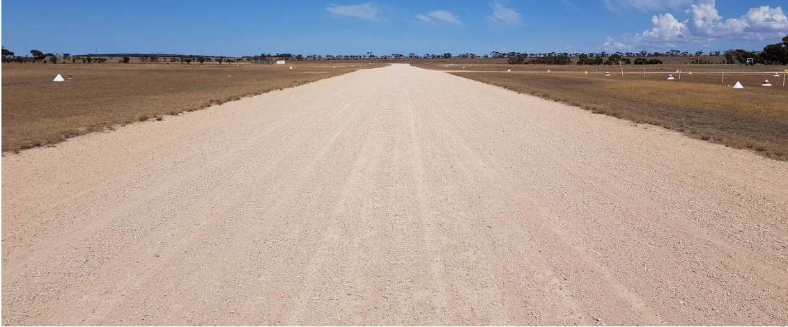
Figure 7 Runway 19 looking south
